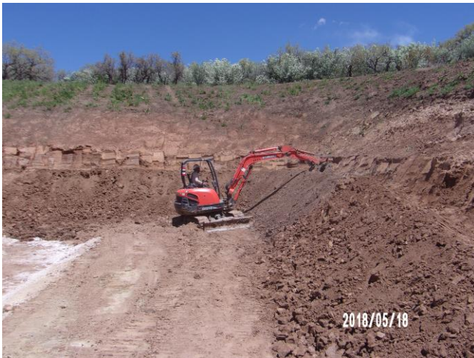
Installing Secondary Berm Mid-Slope
