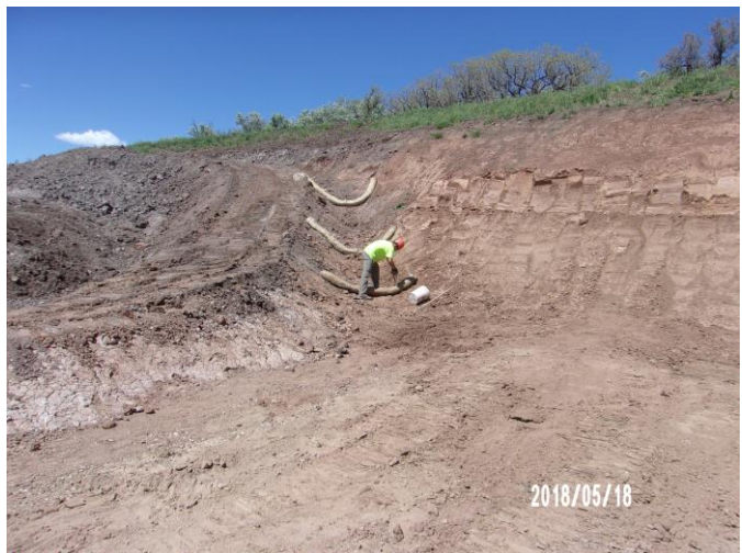
Installing Wattle Checks in Newly Formed Channel
