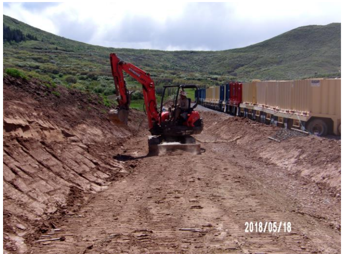
Incorporating Sediment into a Lower Bench
