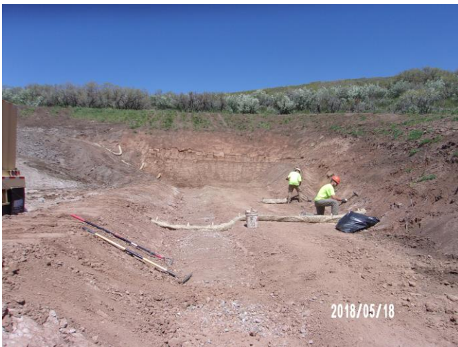
Installing Additional Excelsior Wattle
