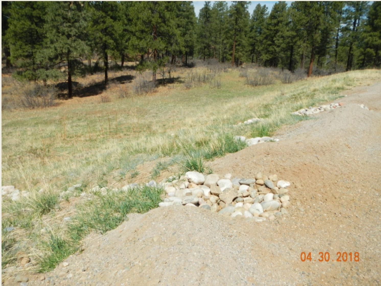
Photo 3. View of cobble run-downs in the western portion of the project area.
