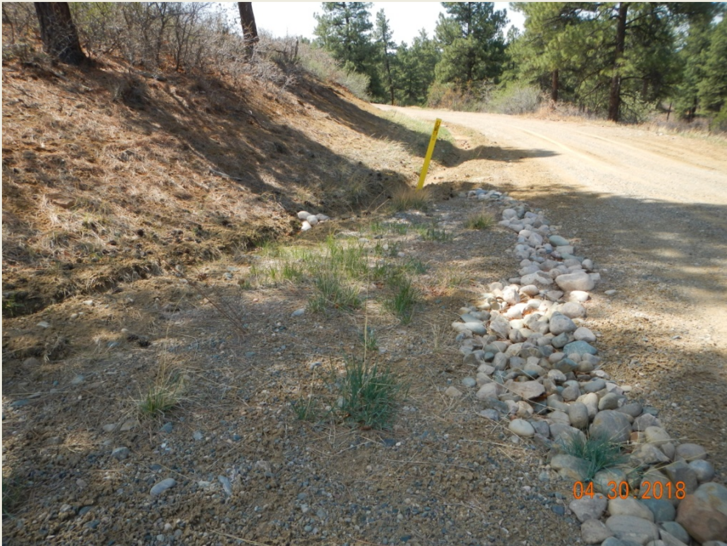
Photo 1. View of cobble armoring and diversion in the southern portion of the project area.
