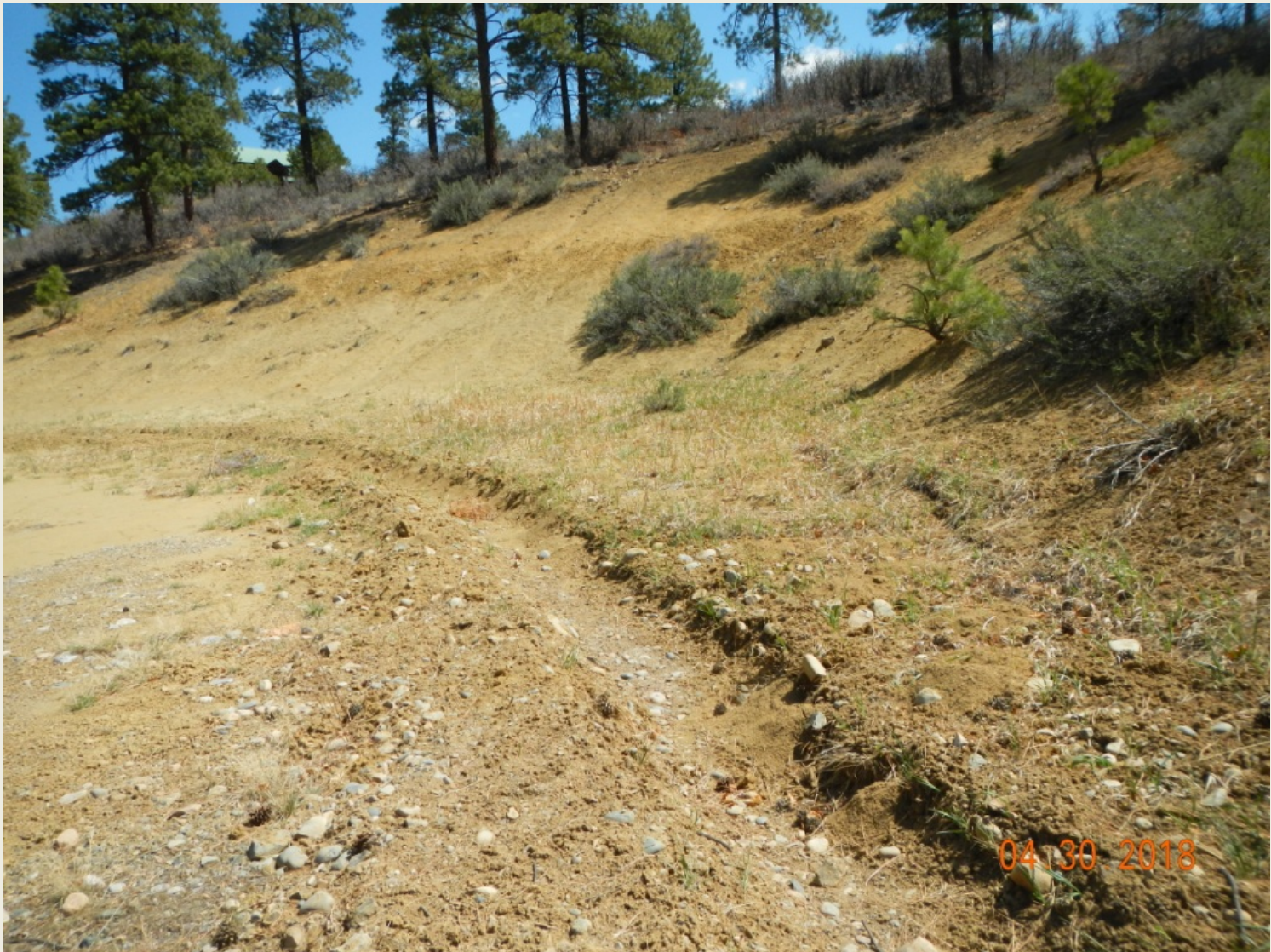
Photo 2. View of recently graded diversion in the southeastern project area.
