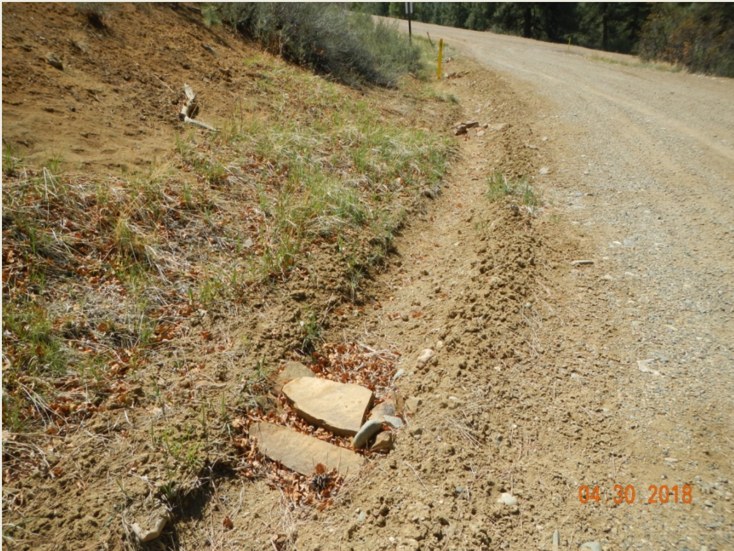
Photo 4. View of rock checks along the access road.
