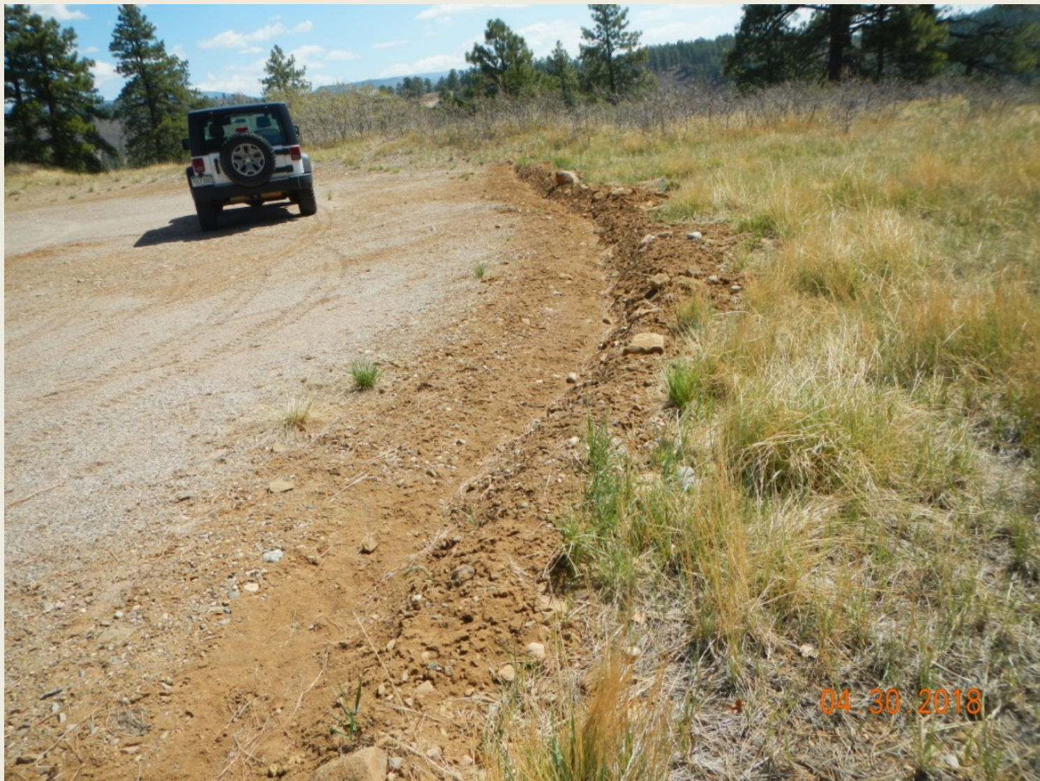
Photo 2. View of area that was recently graded to direct stormwater flows in the southeastern portion of the project area.
