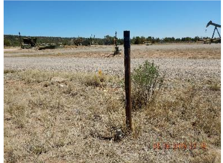
Photo 2: Unused 1" steel riser on N side of access road.
