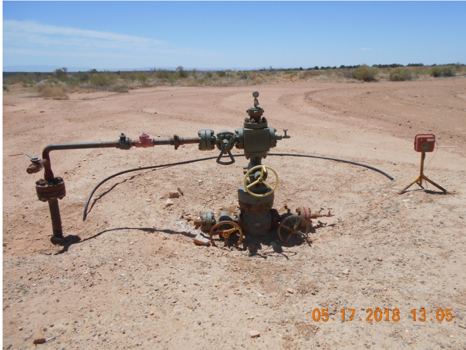
Injection wellhead
