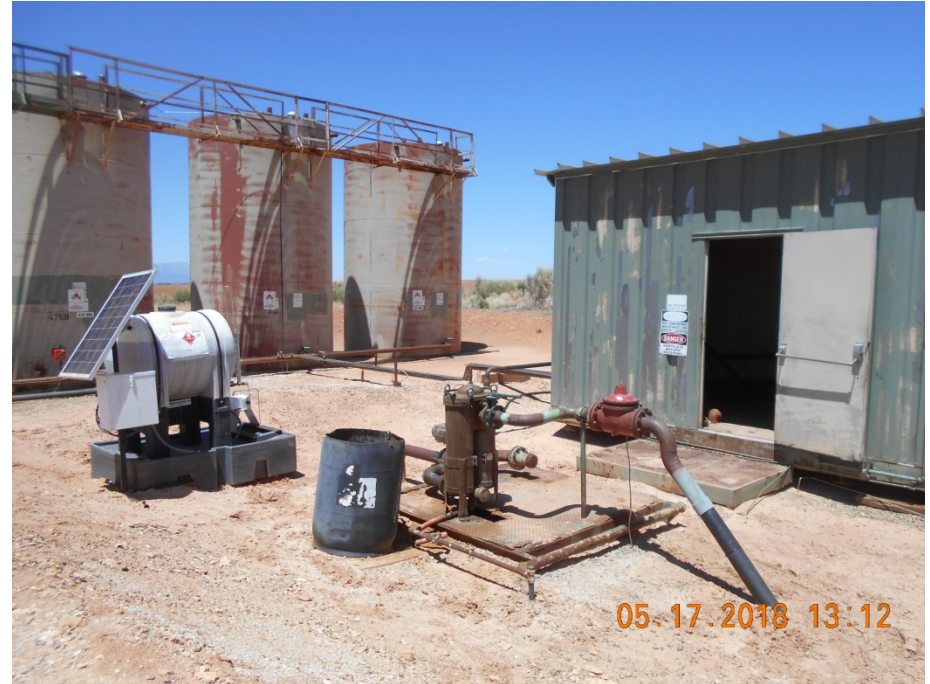
Pump housing, Filter pods and tank battery
