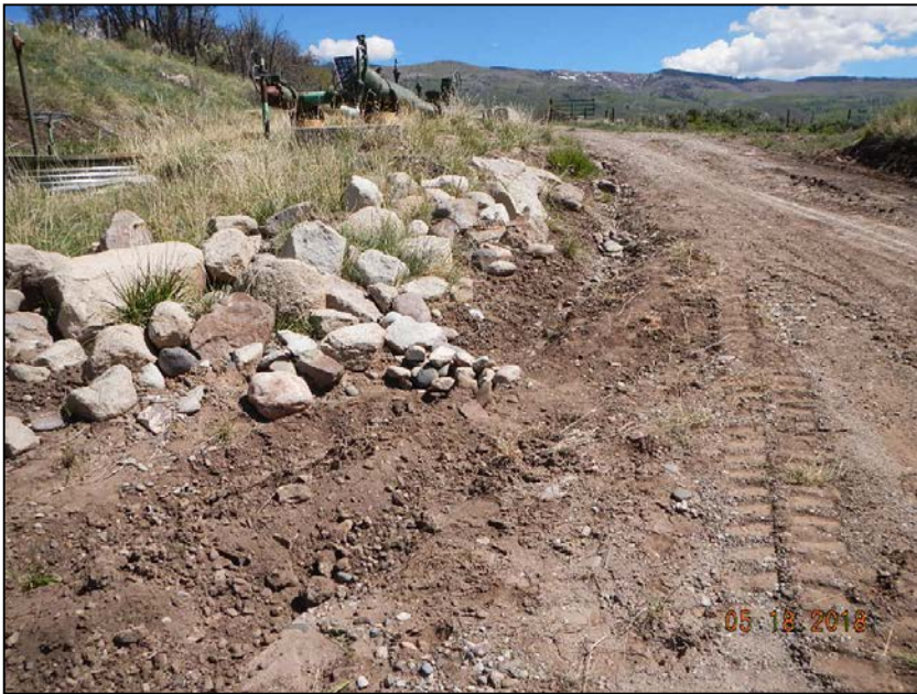
Photo 1. New rock check dams have been installed.
