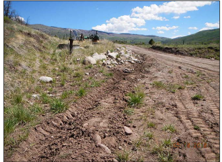
Photo 2. New ditch to prevent run on.
