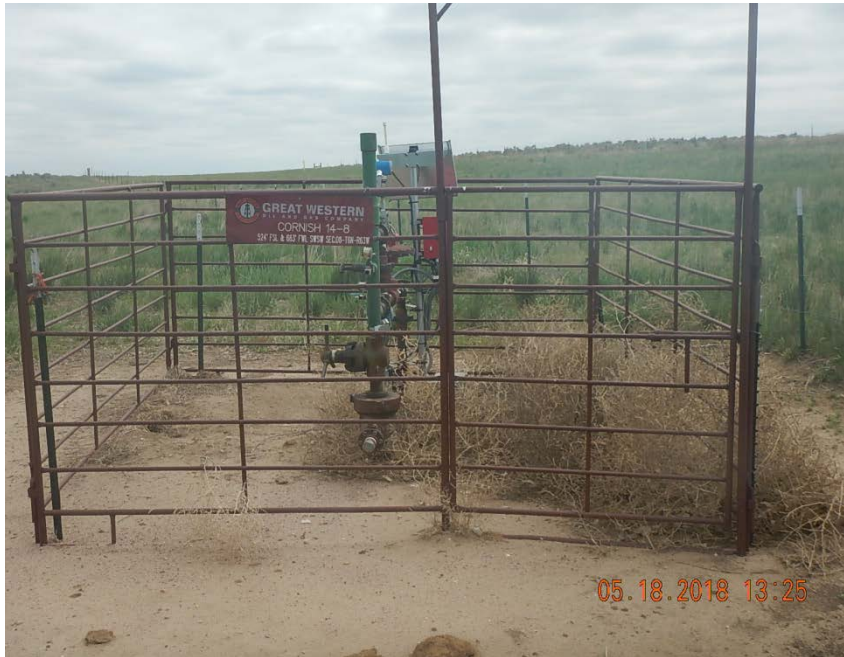
Photo 1: Wellhead, looking S
