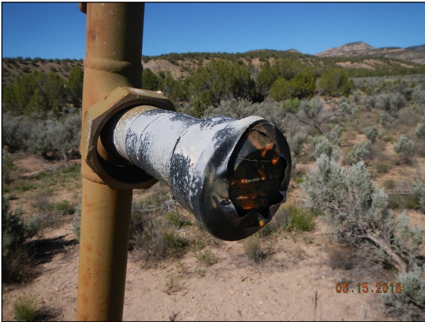
Photo 3. Disconnected flowlines.
