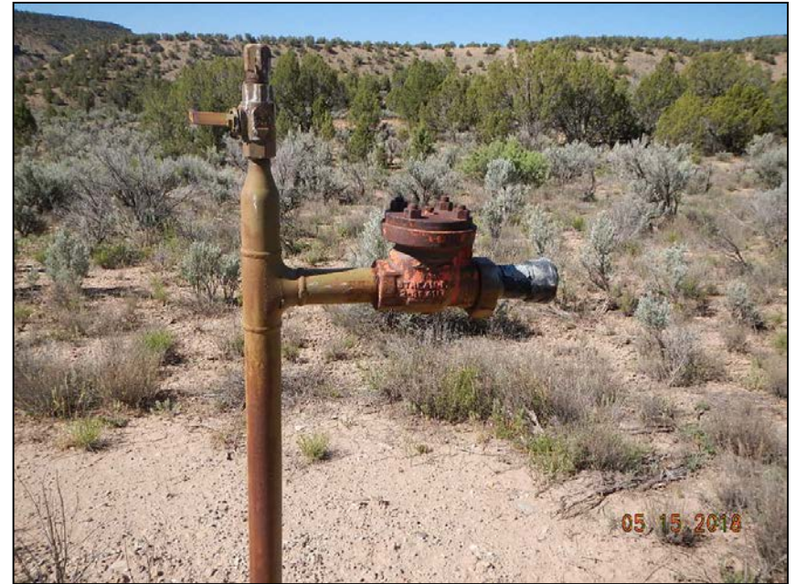
Photo 4. Disconnected flowlines.
