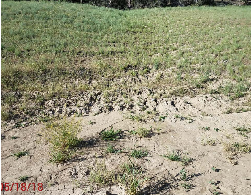
Location Photo #15, Slope erosion on south slope
