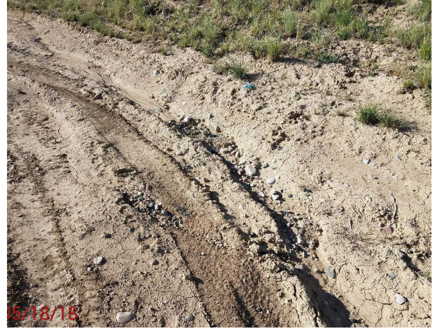
Location Photo # 12, Slope erosion on south slope
