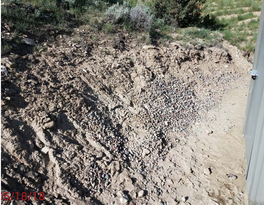
Location Photo #21, slope erosion next to meter run
