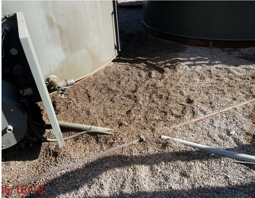
Location Photo # 3, Staining in Tank Battery containment
