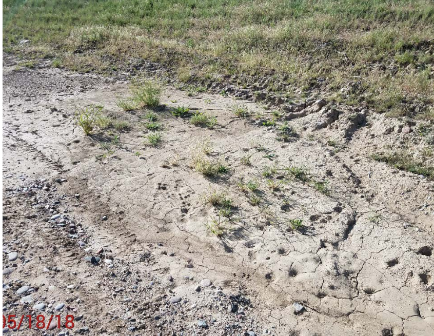
Location Photo #13, Slope erosion on south slope
