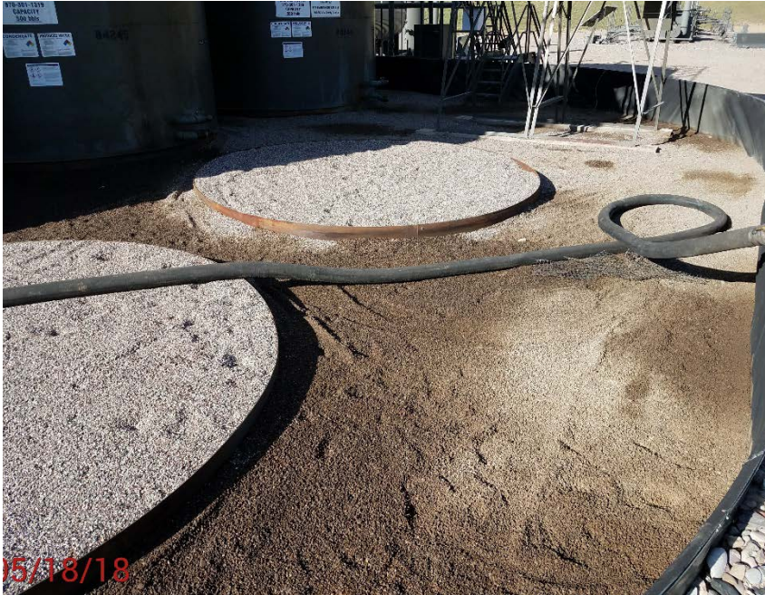
Location Photo #7, Staining in Tank Battery containment
