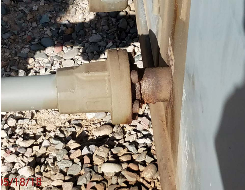
Location Photo #9, Leaking liquid line from back of separator
