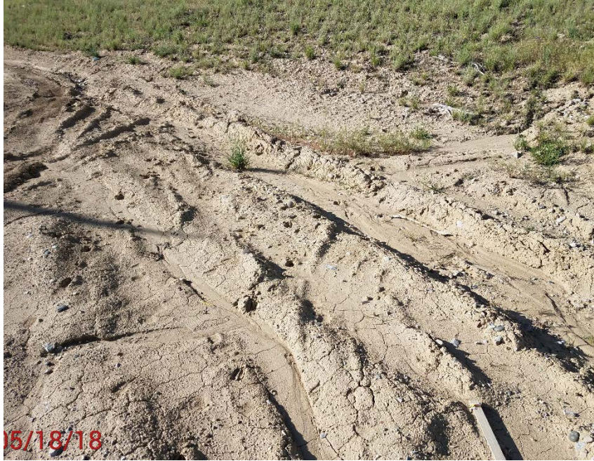
Location Photo #11, Slope erosion on south slope
