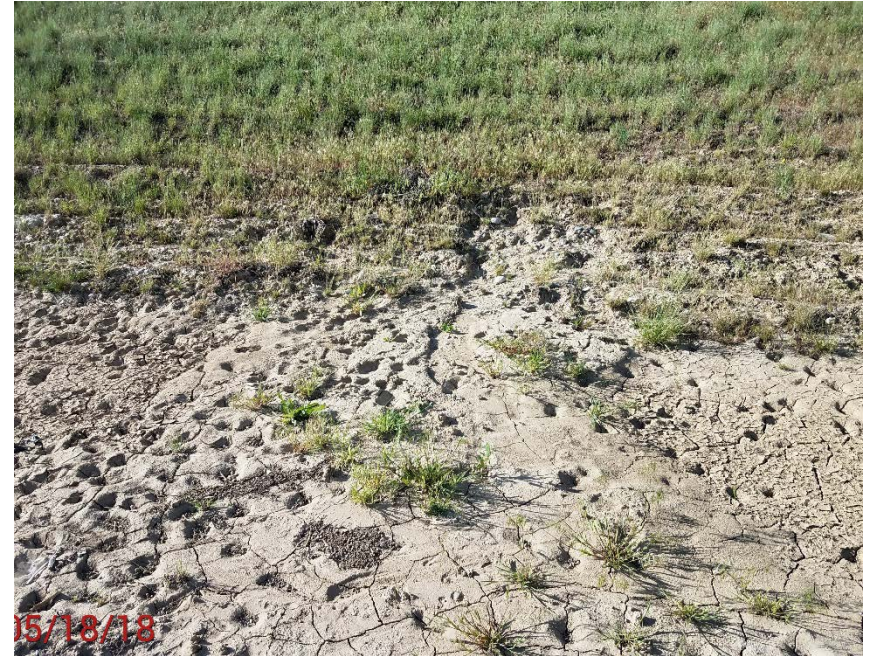
Location Photo # 16, Slope erosion on south slope
