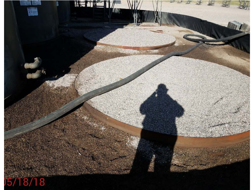
Location Photo # 6, Staining in Tank Battery containment
