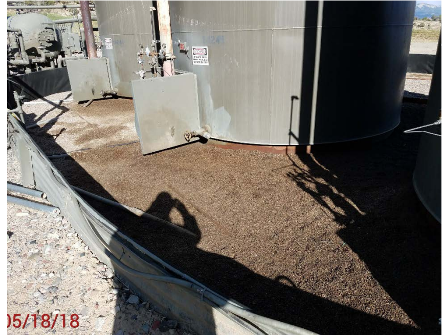
Location Photo # 4, Staining in Tank Battery containment
