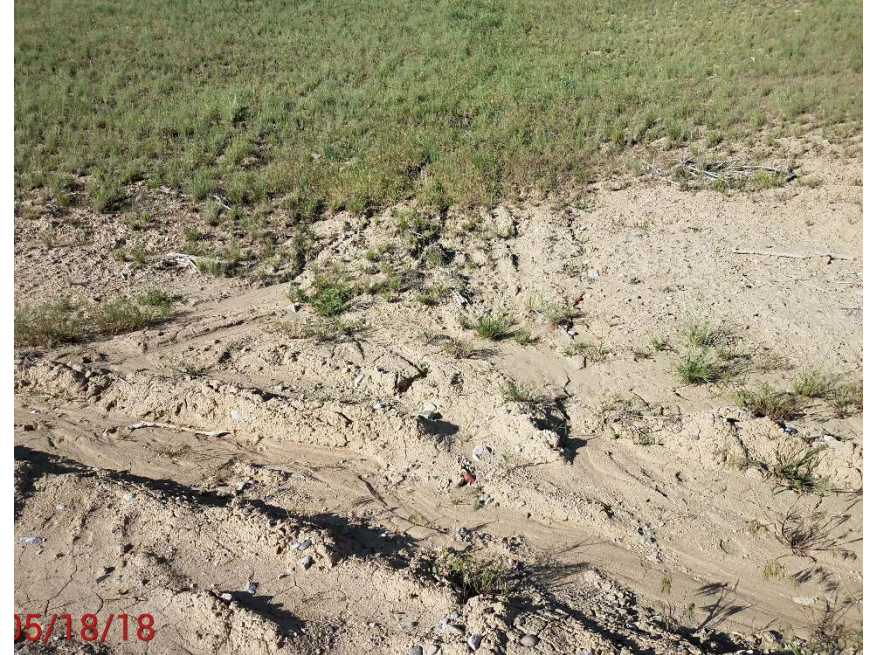
Location Photo # 10, Slope erosion on south slope
