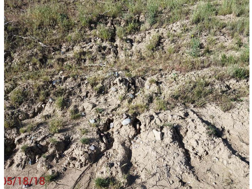
Location Photo # 14, Slope erosion on south slope
