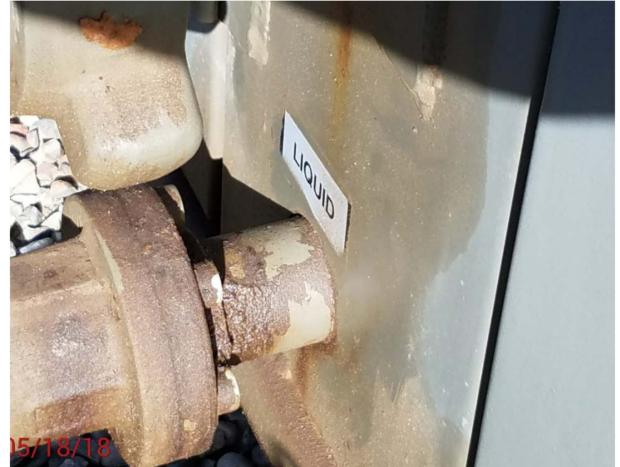
Location Photo #8, Leaking liquid line from back of separator
