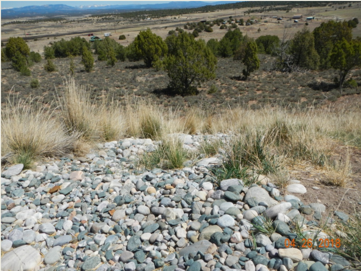
Photo 4. View of cobble run-down within the northeastern portion of the project area.
