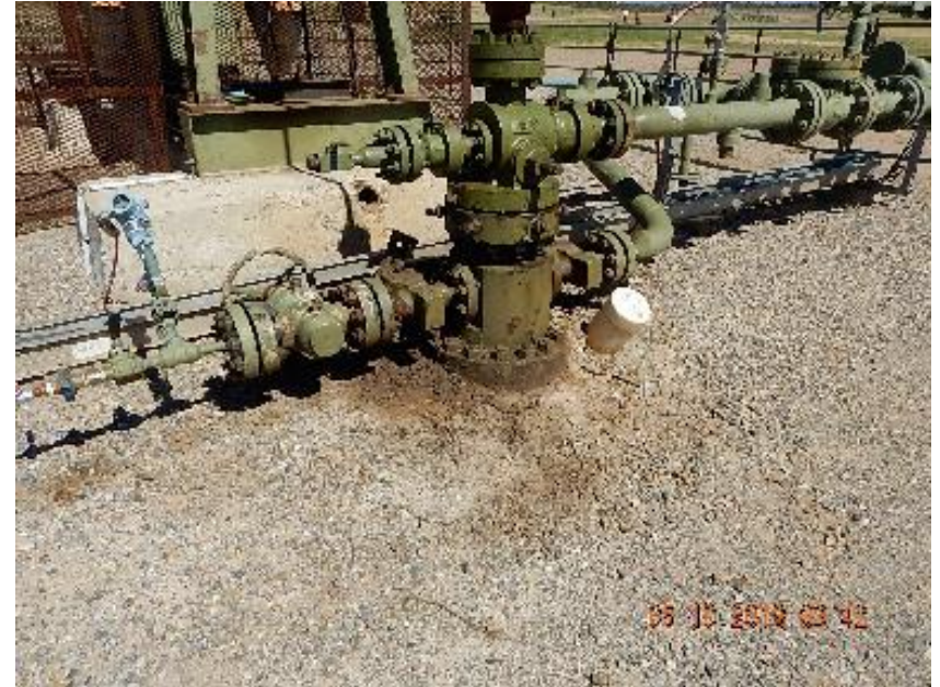
Photo 2: Impacted soil and gravel around wellhead.
