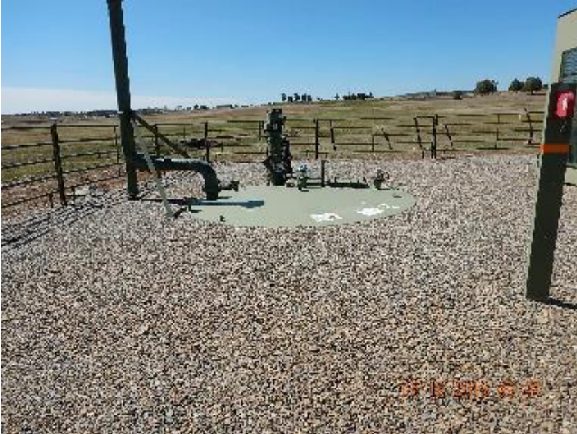
Photo 3: Labels on production tank top.
