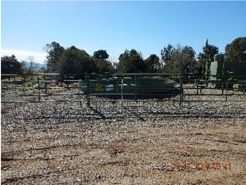
Photo 5: NFPA label not visible from outside containment ring.
