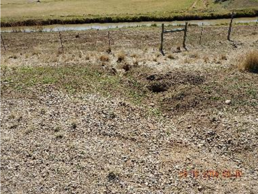
Photo 3: Erosion channel in NE corner.
