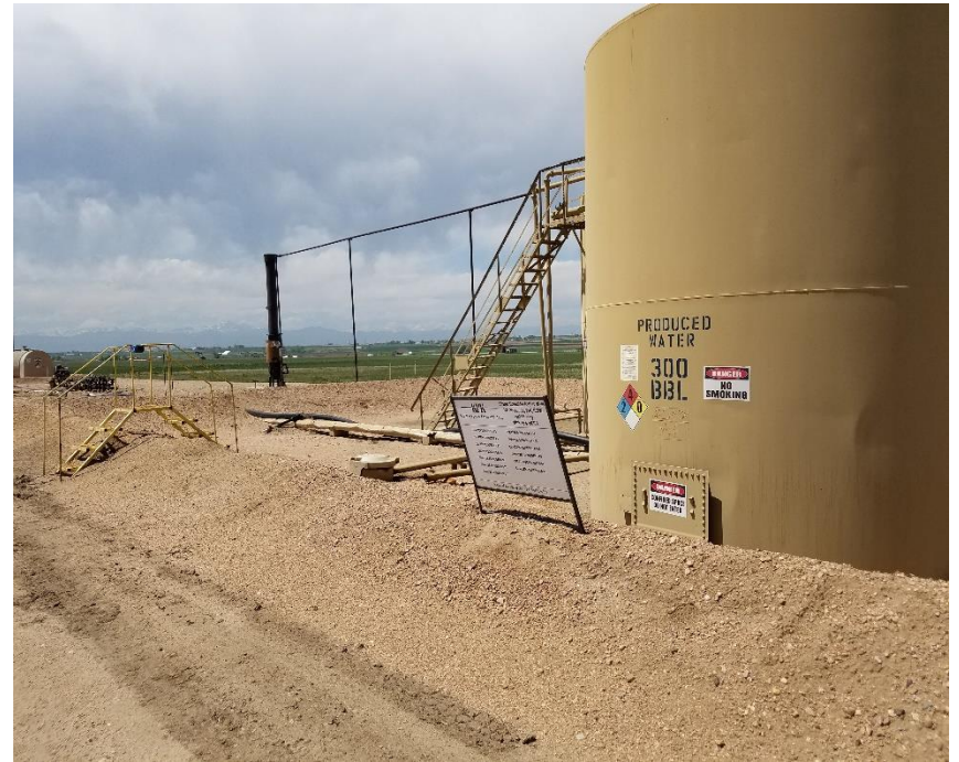
Photo 2. Tank battery
