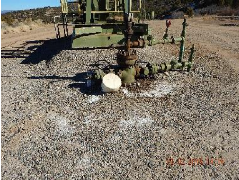
Photo 5: Impacted soil around wellhead previous inspection.
