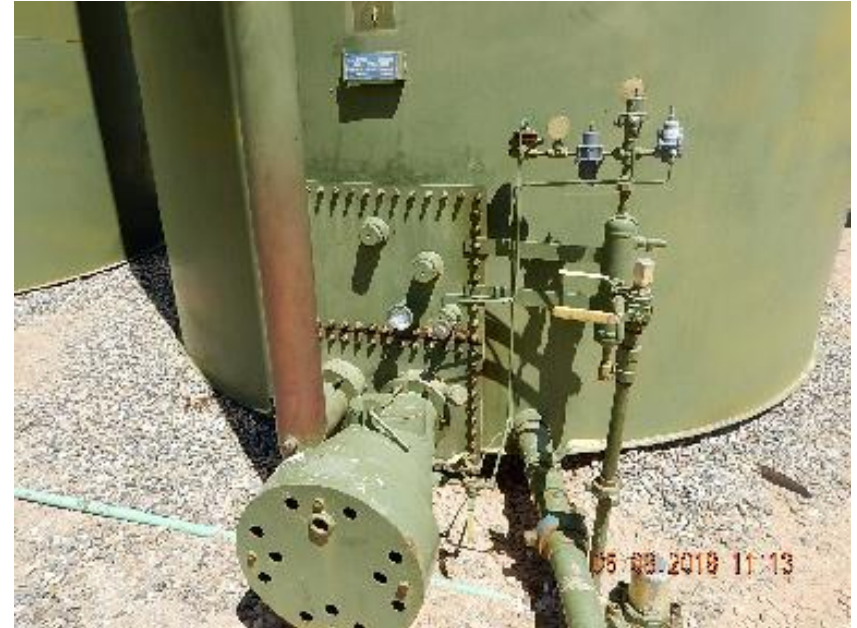
Photo 10: Tank heater tube hatch.
