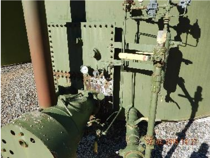
Photo 9: Mineral deposits on tank heater tube hatch previous inspection.
