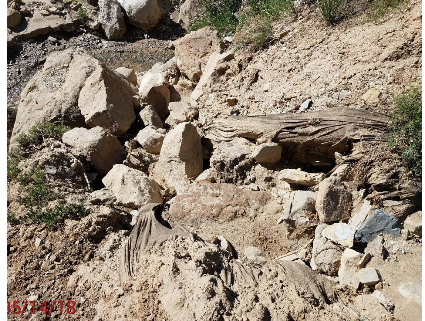
Location Photo #19, Erosion on down hill side of retention pond
