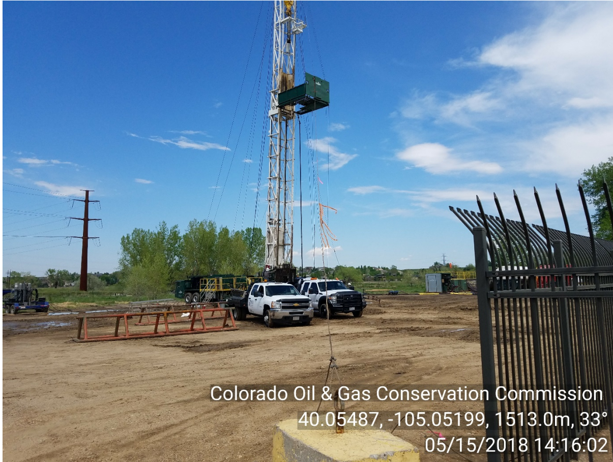
Swabco rig #18, rigging up to plug & abandon Sosa 12-18
