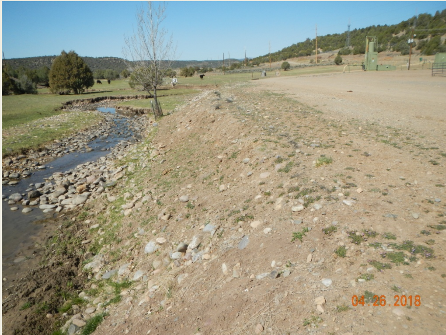
Photo 4. View of the southern portion of the project area from the southeastern corner facing westward. No significant erosion observed; however, this area needs to be carefully monitored or more robust stormwater controls installed.
