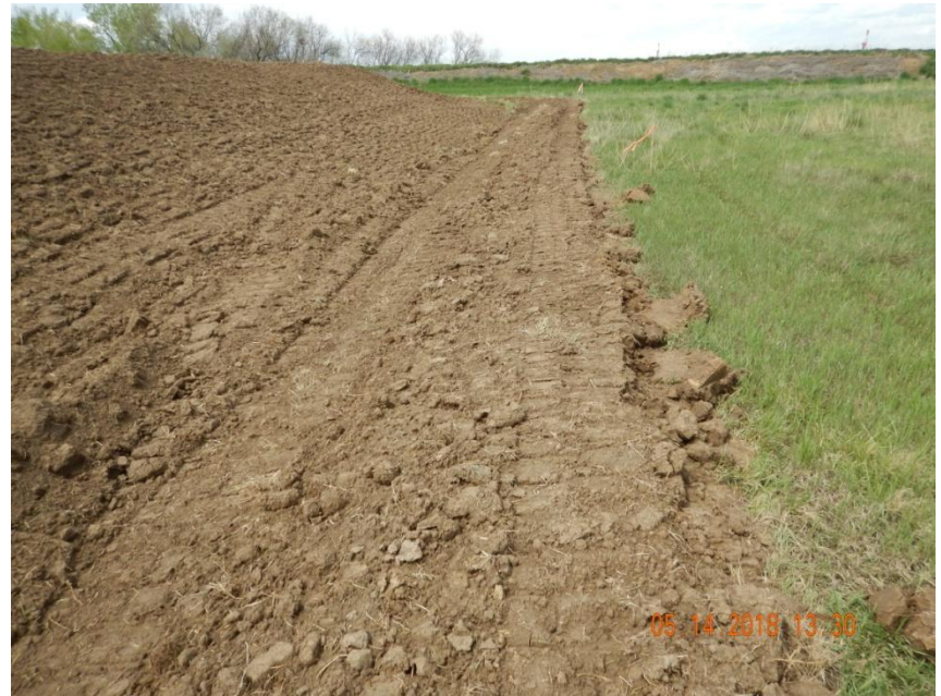
Photo 4. Photo taken from the northeast perimeter of the location, facing North. Ditch BMP has been filled in from construction operations and needs maintenance. Topsoil has been stockpiled and temporarily stabilized with equipment tracking along the eastern perimeter of the location.
