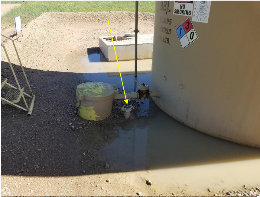
Photo 3. Unmarked riser near crude oil tank load out.
