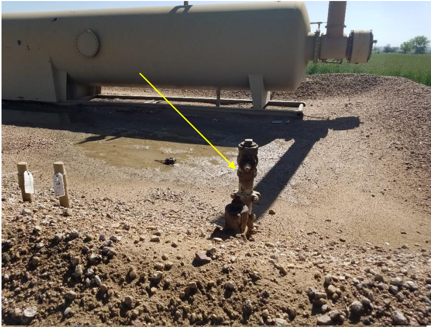
Photo 5. Unmarked riser near heated treater
