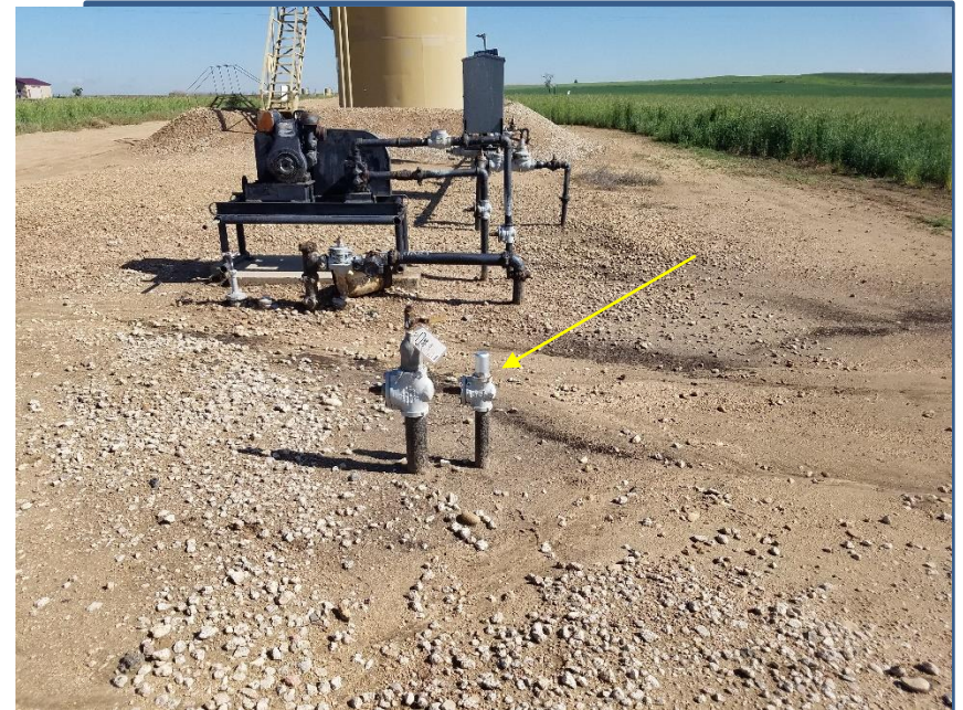
Photo 4. Unmarked riser near transfer pump
