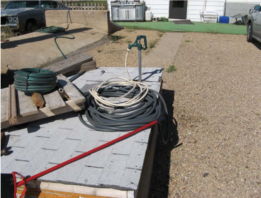
Photo 5 – View of hydrant at well vault/sump for domestic water well permit no. 202929A which supplies the residence. Water sample collected from hydrant in photo.
