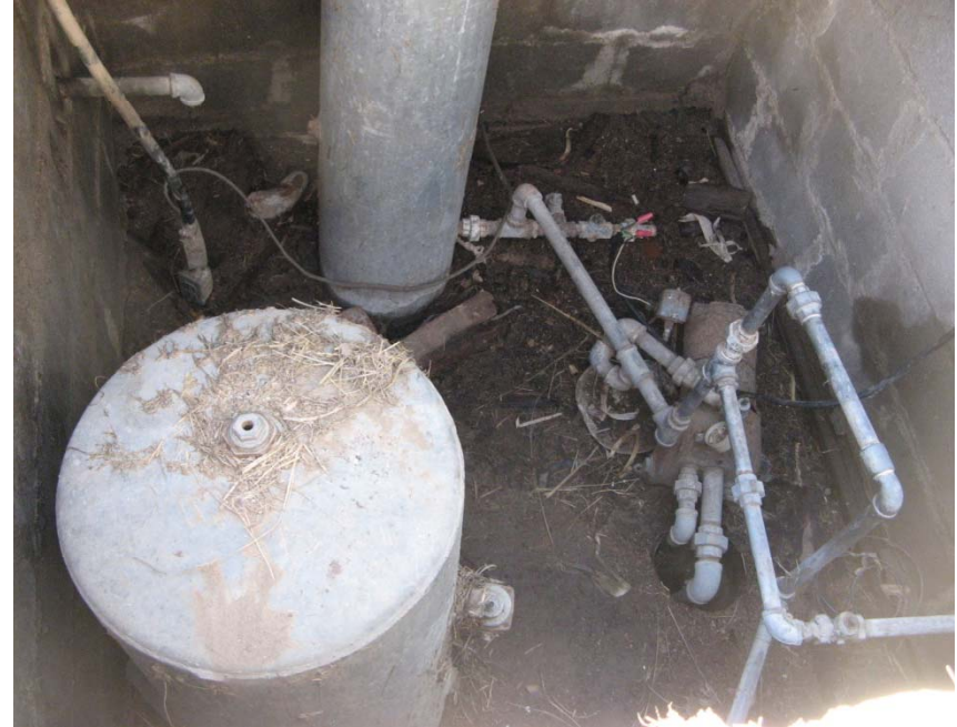
Photo 2 – Second view of domestic water well vault/sump for well permit no. 276778 showing pressure tanks.
