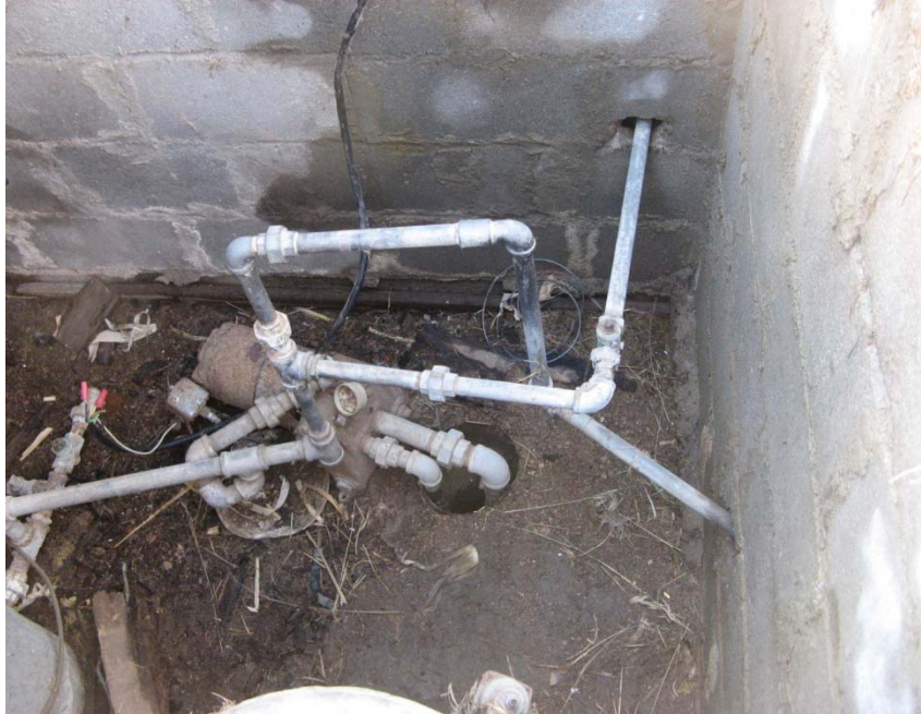
Photo 1 – View of domestic water well vault/sump for water well permit no. 276778. Well casing is open hole in sump. Motor has seized and a sample was not collected.
