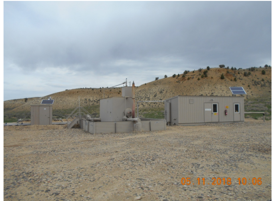
Pump housing and Separator and Meter housing
