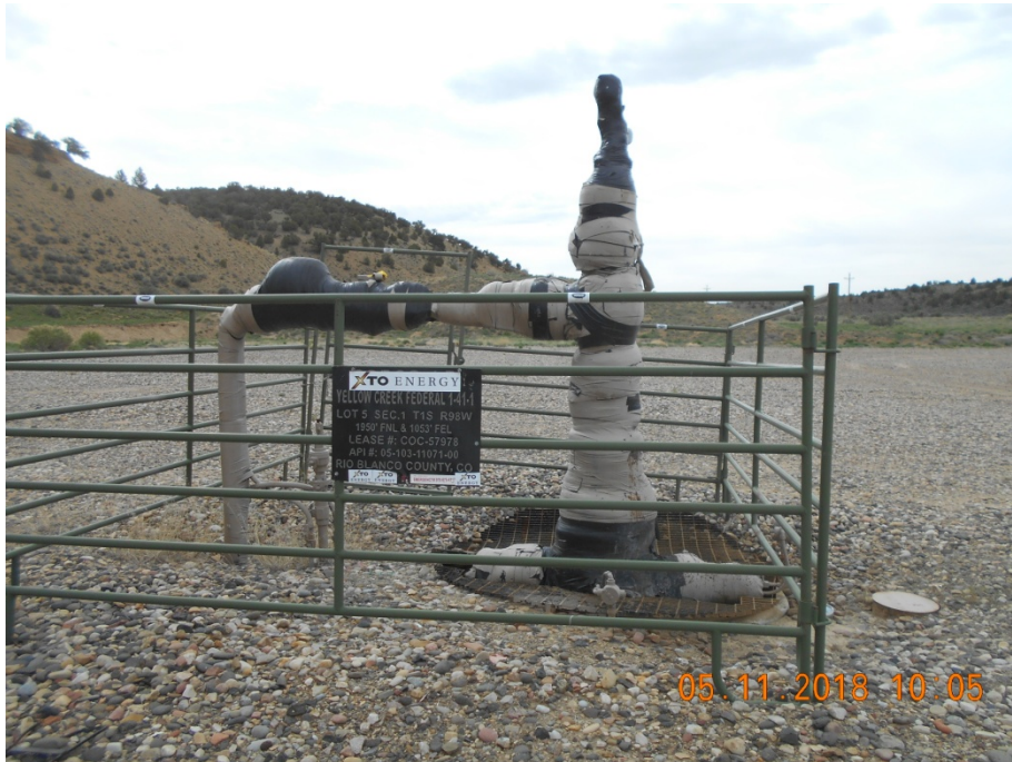
Injection wellhead with fencing and sign
