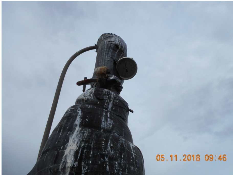
Tubing gauge on wellhead
