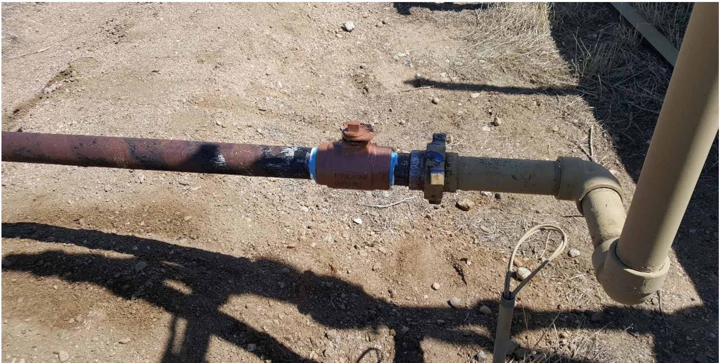
Figure #2 Stained soil was removed, the valve was replaced
