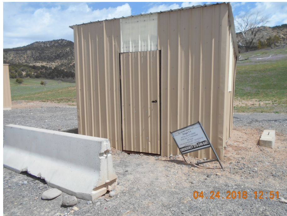
Injection wellhead housing with sign
