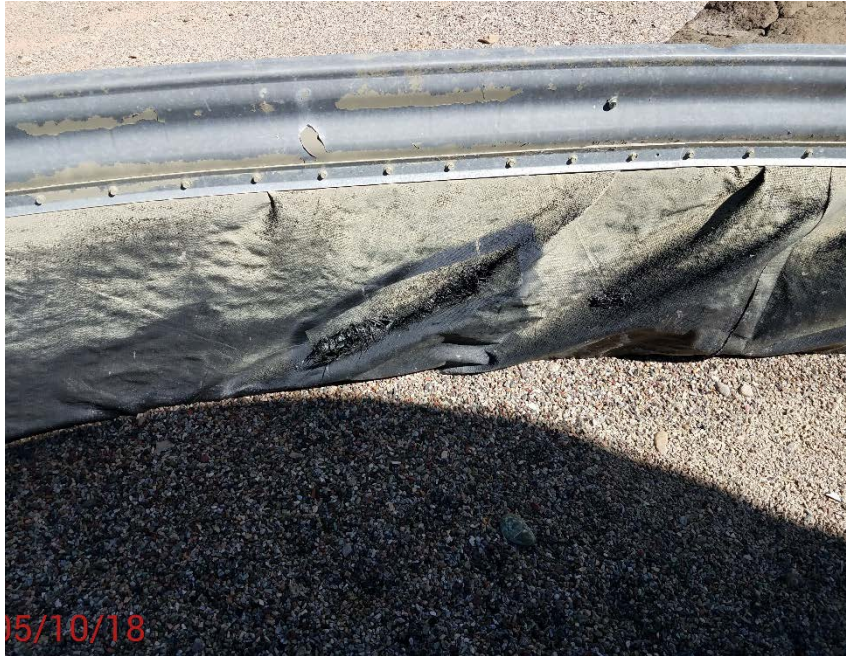
Location photo # 3, Holes in containment liner
