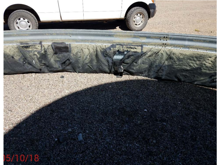
Location photo # 2, Holes in containment liner
