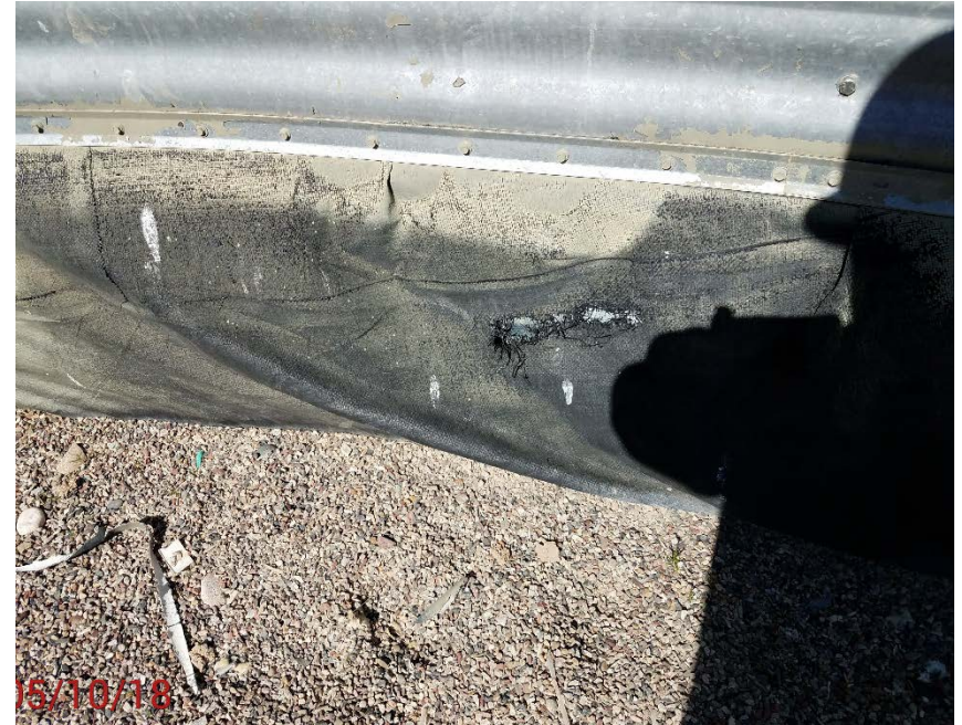
Location photo # 4, Holes in containment liner
