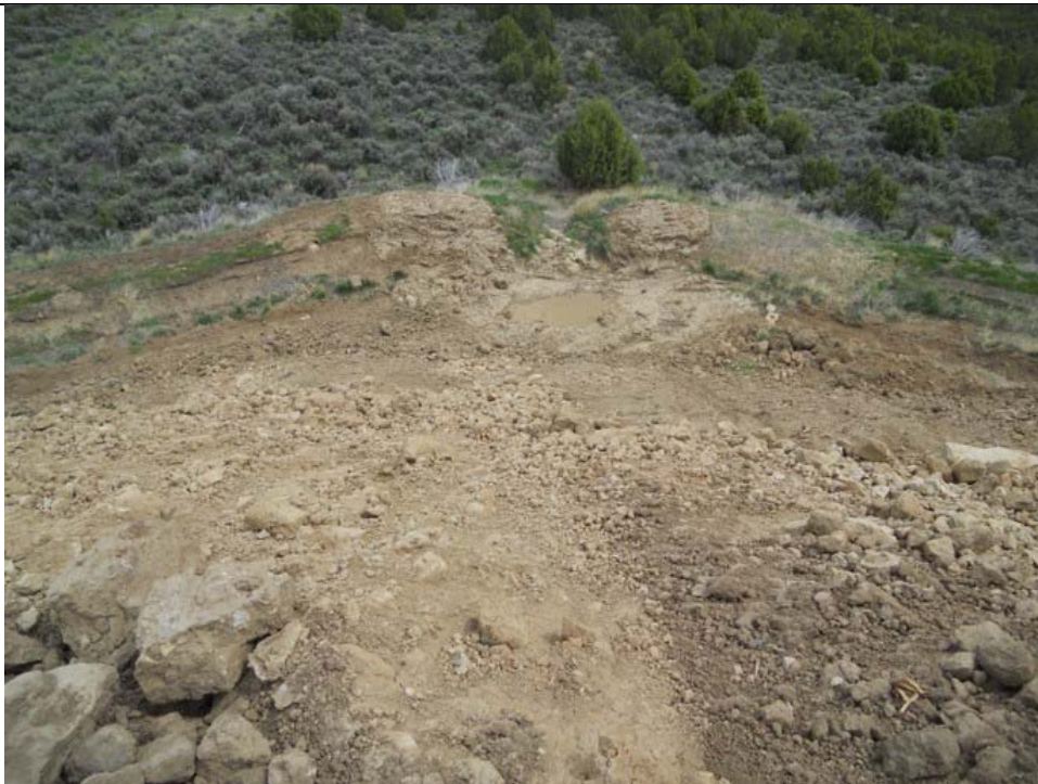
Photograph 7: NE Sediment Trap (2.25-acre capacity)
