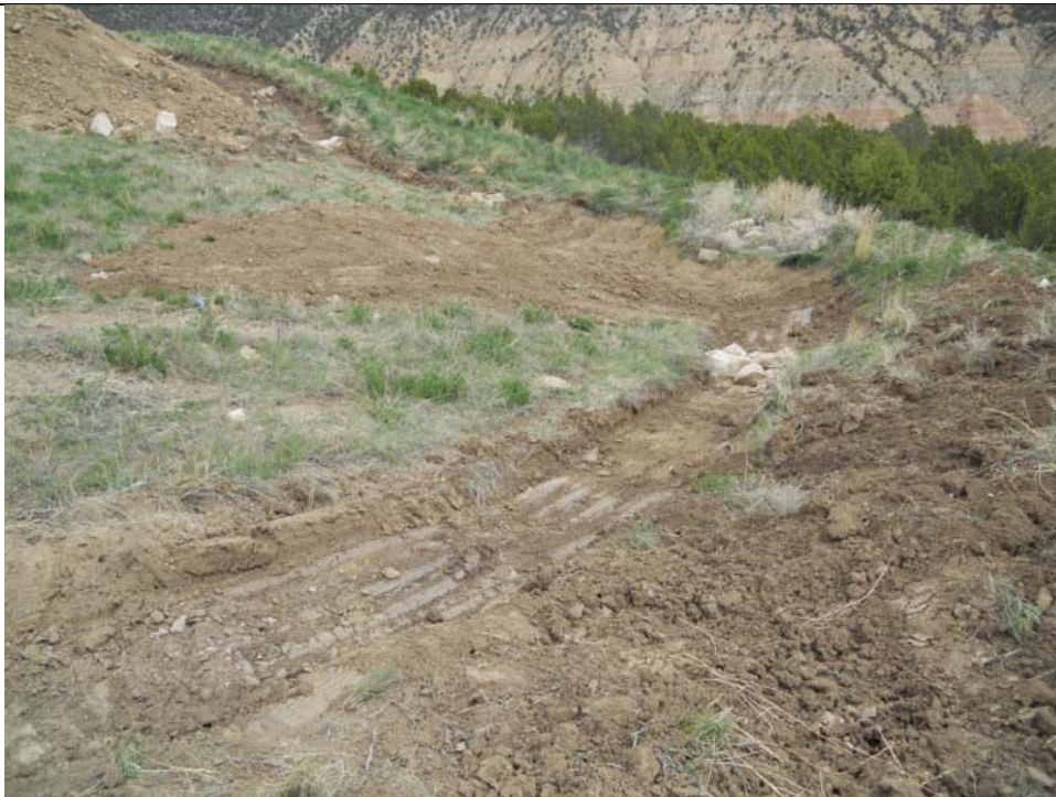
Photograph 1: SE Sediment Trap (3.25-acre capacity)
