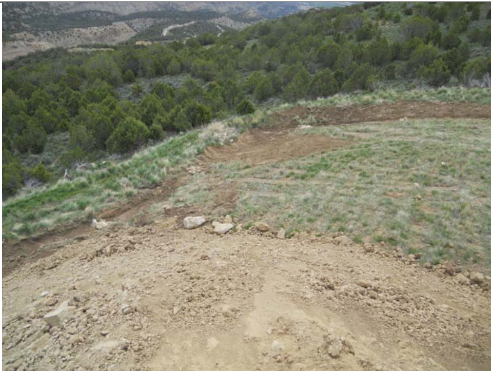
Photograph 5: SE Sediment Trap (3.25-acre capacity)/Top Soil Berm
