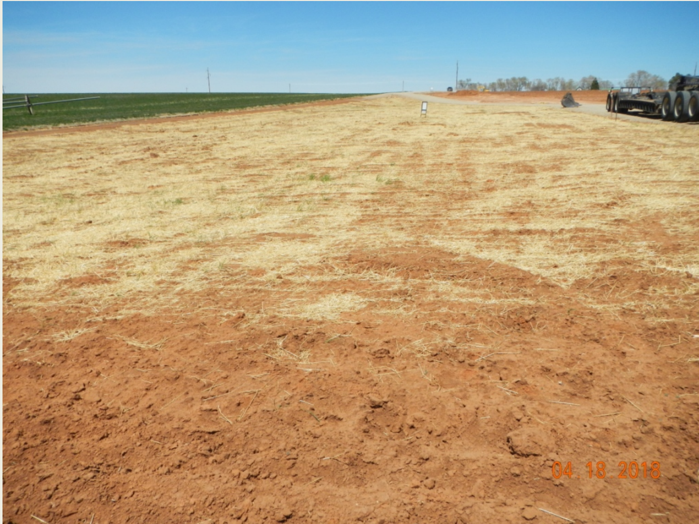
Photo 3. View of the western portion of the project area from the southwestern corner facing northward. Western portion of project area is in process of being revegetated. Straw mulch and seedlings observed.
