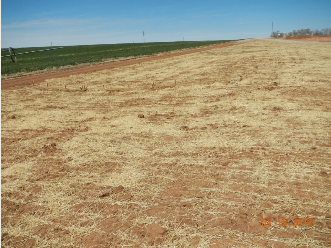
Photo 4. Another view of western interim reclamation area and straw wattles in shallow swale along the western edge of the project area. Appear to be functioning.
