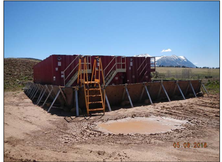
Photo 2. Temporary tanks and containment.
