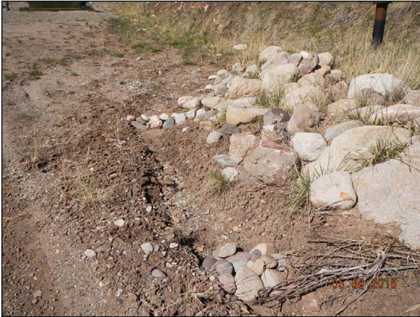
Photo 5. Stormwater and sediment continue to run on location.
