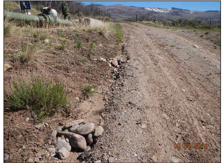
Photo 4. Check dams have failed.
