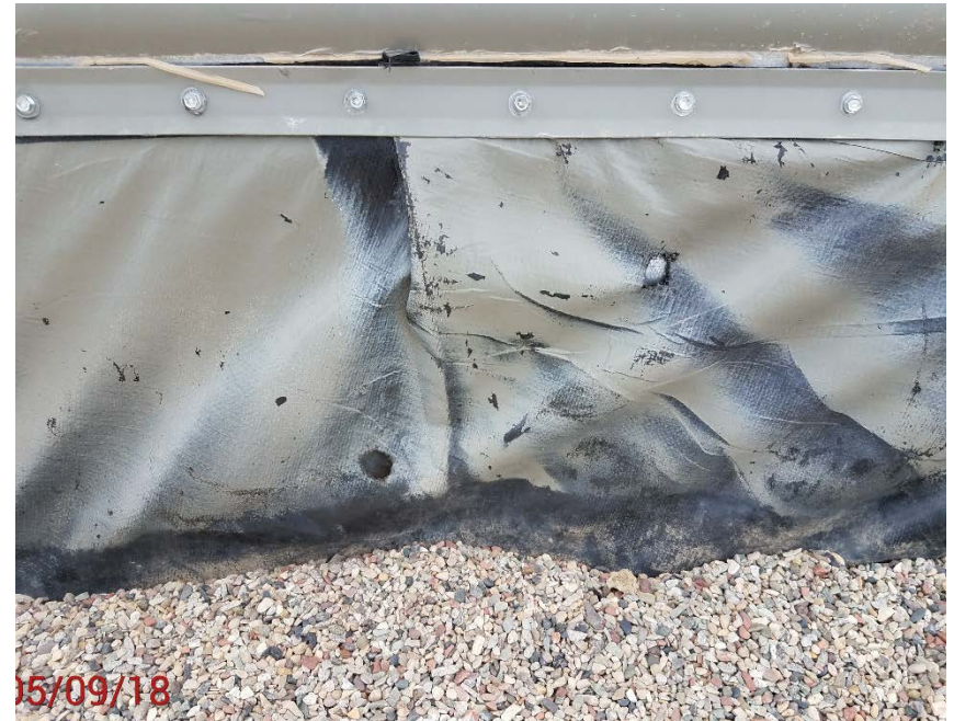
Location photo # 6, Holes in tank battery liner
