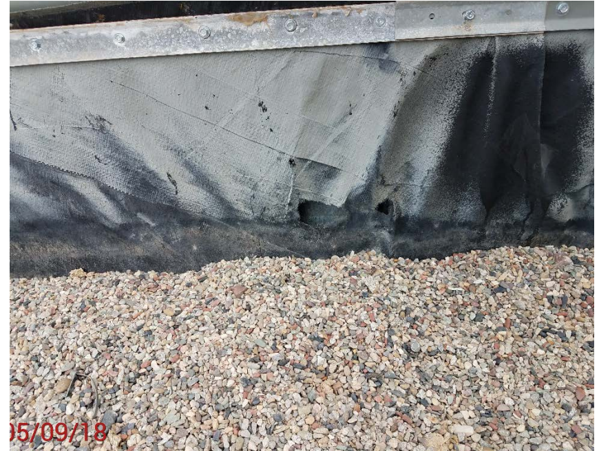
Location photo # 8, Holes in tank battery liner
