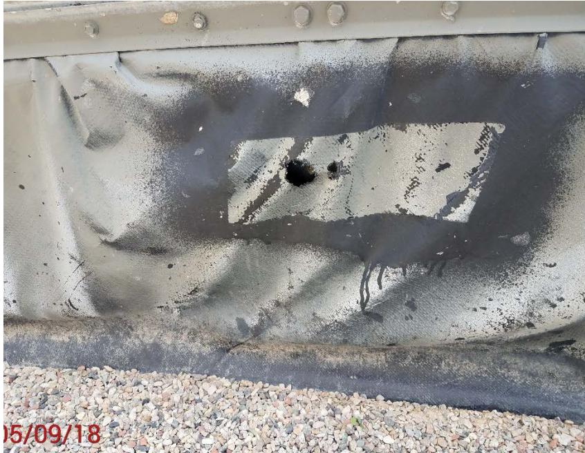
Location photo # 1 Holes in tank battery liner
