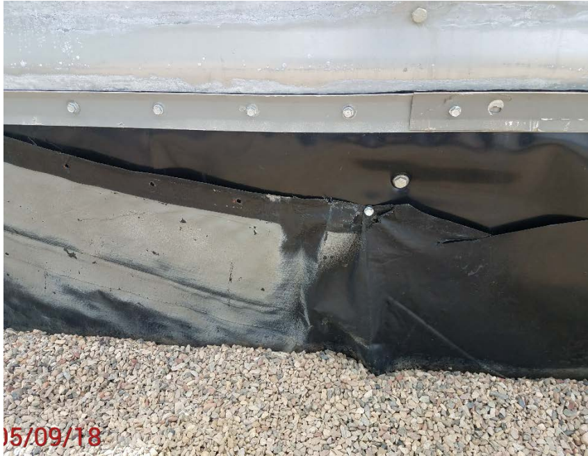
Location photo # 7, Holes in tank battery liner
