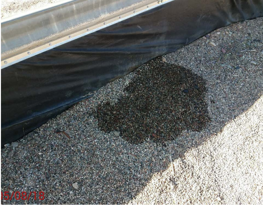
Location photo # 9, stained rock in tank battery liner
