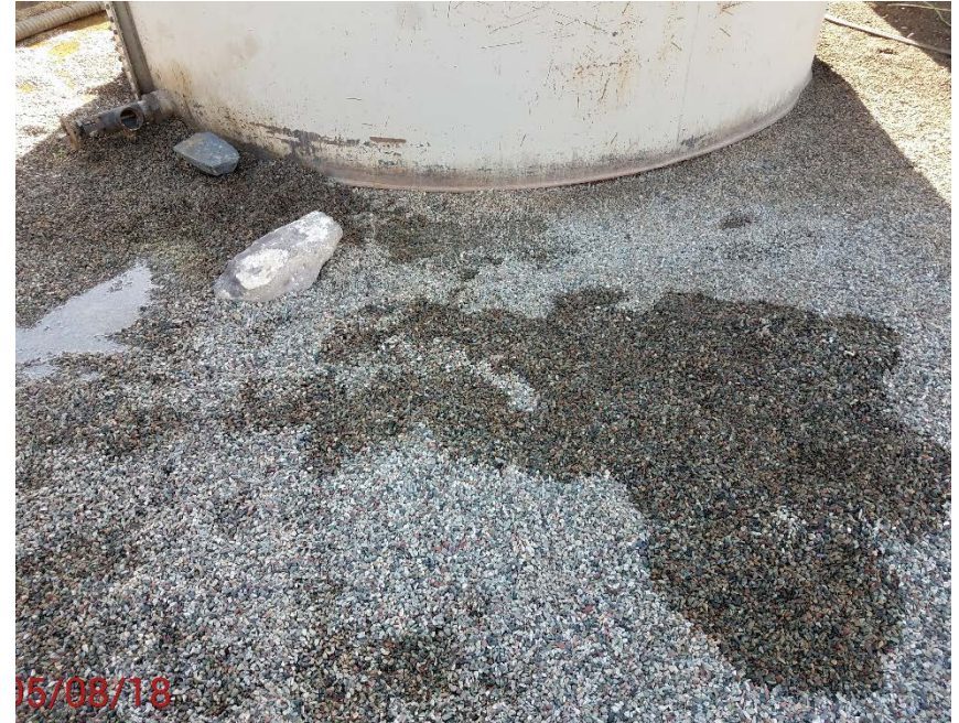
Location photo # 6, stained rock in tank battery liner
