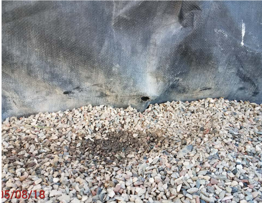
Location photo # 3, holes tank battery liner
