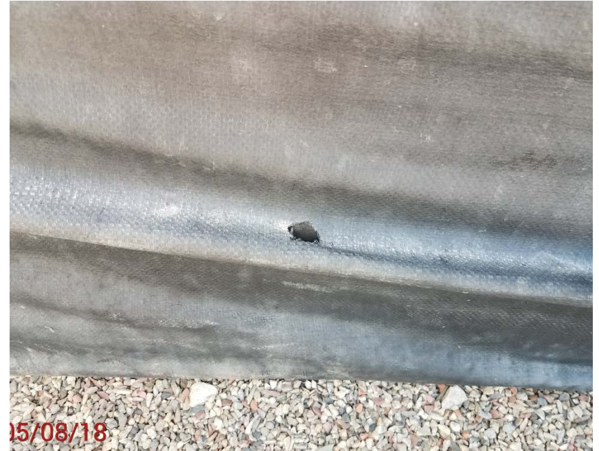
Location photo # 4, holes tank battery liner
