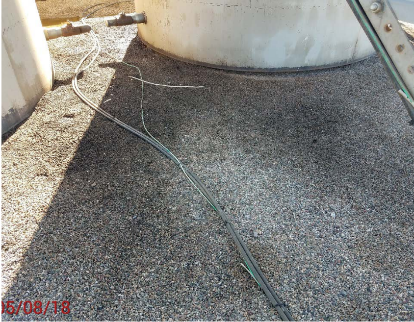
Location photo # 7, stained rock in tank battery liner
