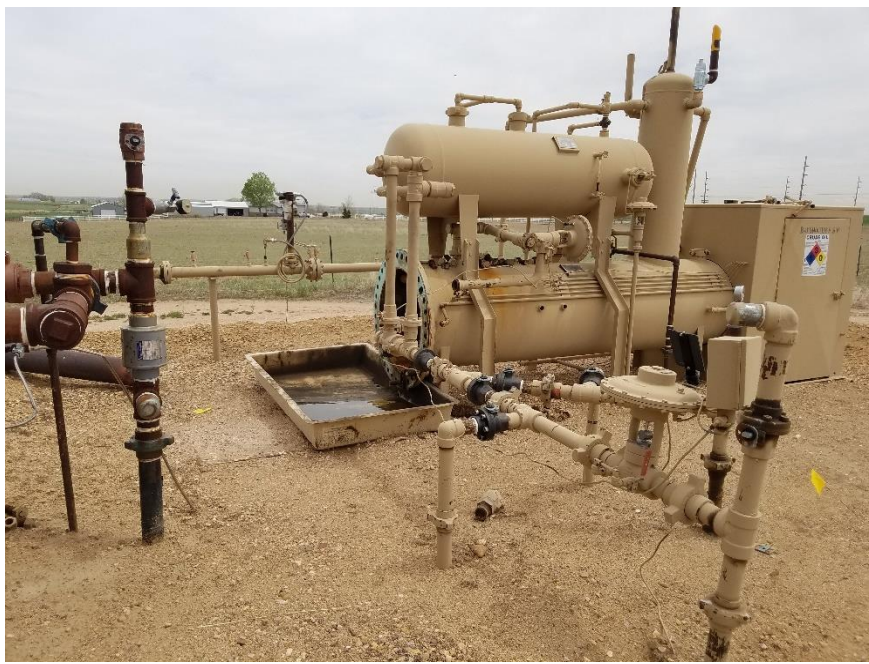
Photo 3. Heated separator
