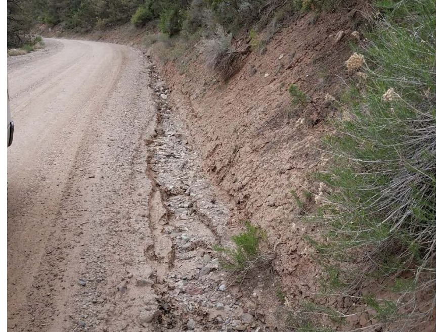
Location photo # 19, Storm water issue on access road
