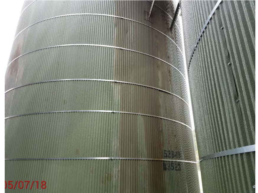
Location photo # 12, Oily residue on tank
