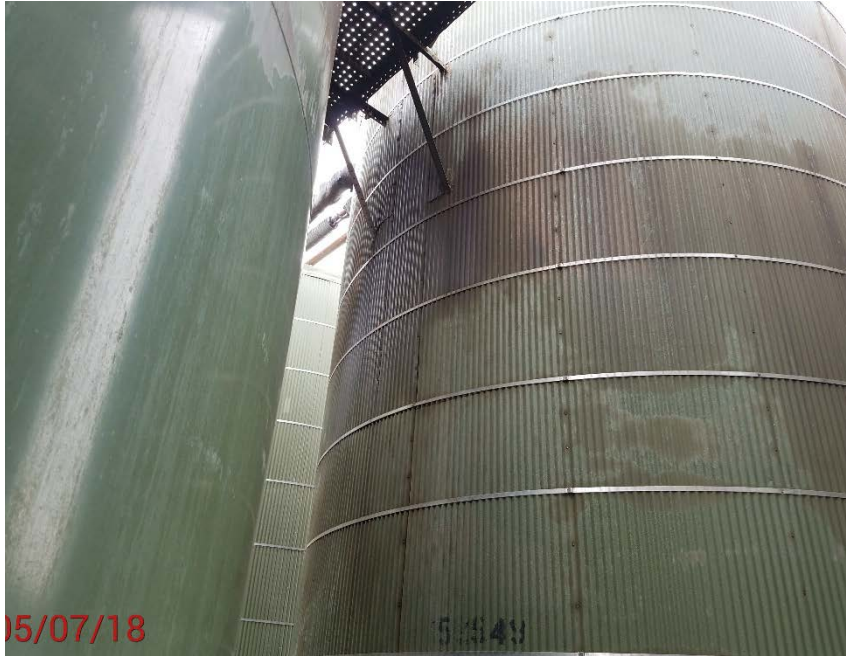
Location photo # 11, oily residue on tank
