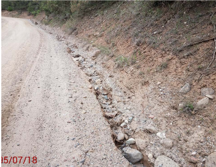
Location photo # 16, Storm water issue on access road
