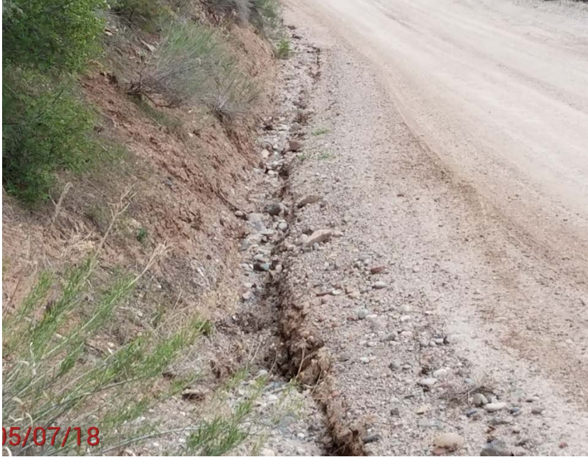
Location photo # 18, Storm water issue on access road
