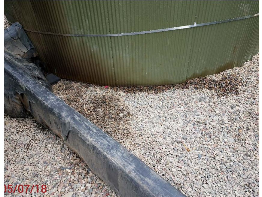
Location photo # 10, stained rock in tank battery containment
