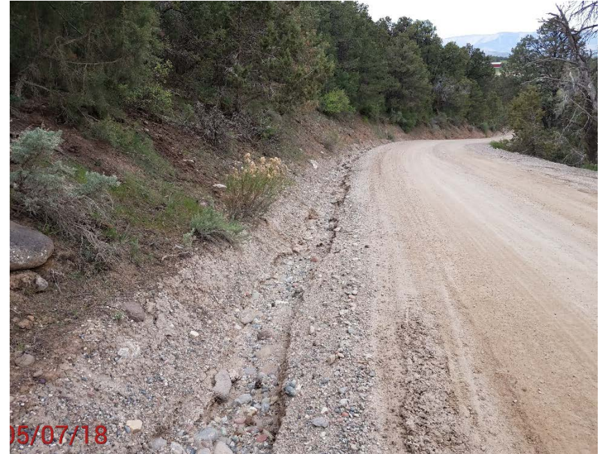
Location photo # 15, Storm water issue on access road
