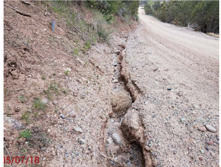
Location photo # 17, Storm water issue on access road
