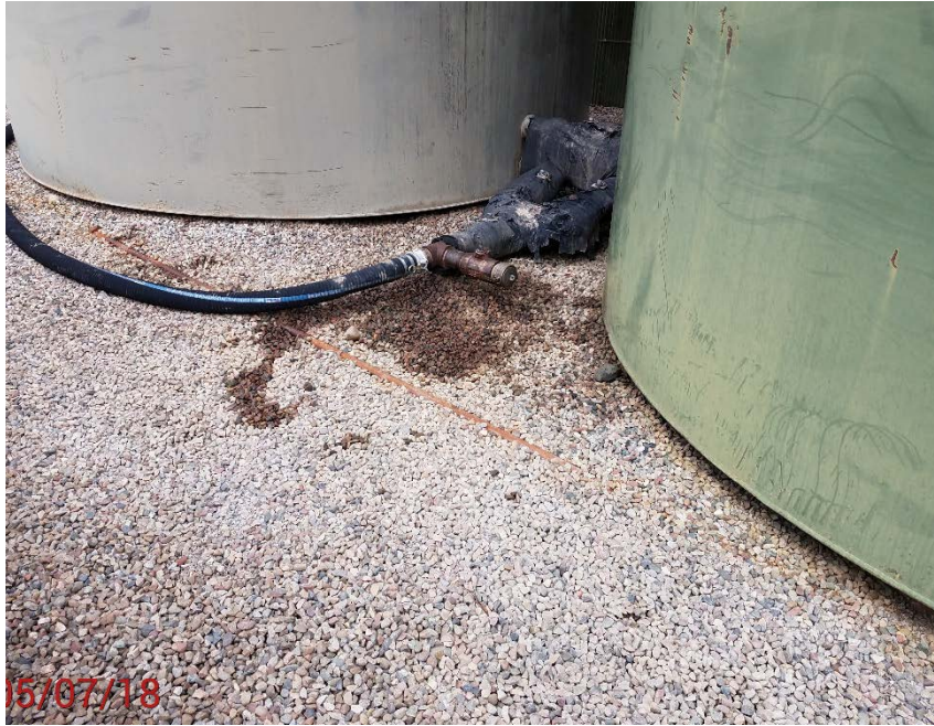
Location photo # 7, Stained rock in tank battery containment
