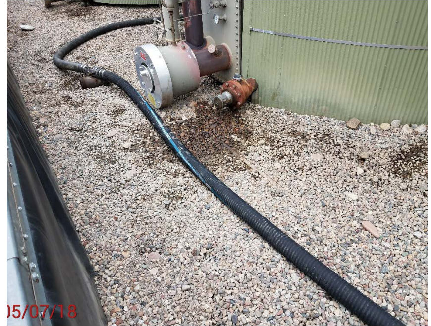
Location photo # 8, stained rock in tank battery containment
