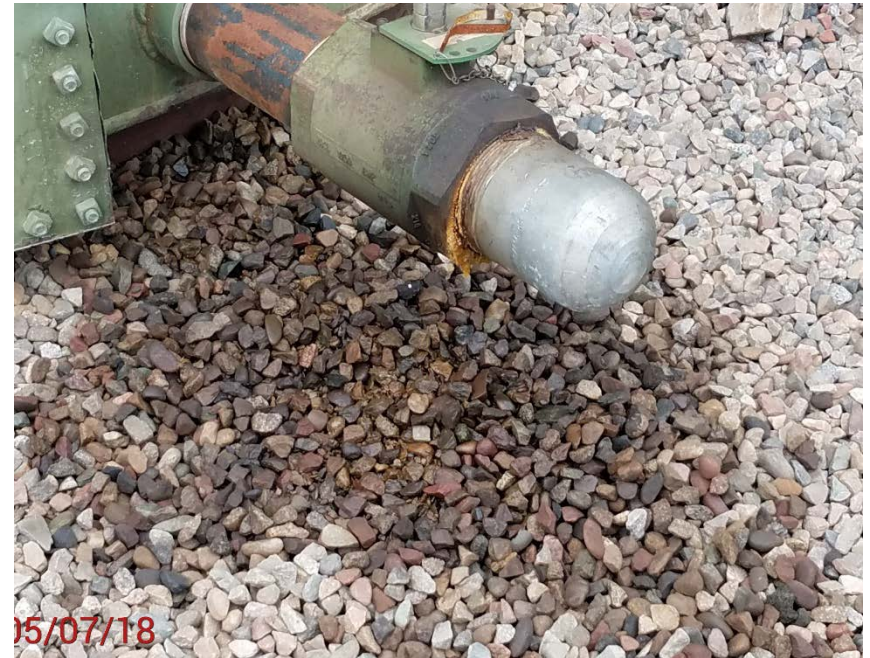
Location photo #6, Stained rock in tank battery containment.
