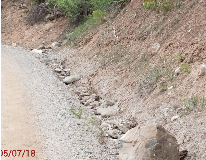
Location photo # 14, Storm water issue on access road
