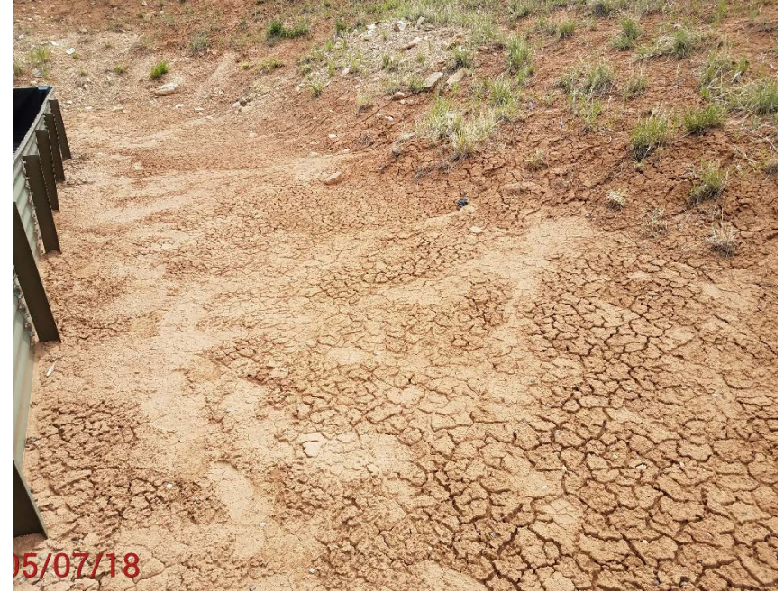
Location photo #6 storm water erosion on SE corner of Tank Battery
