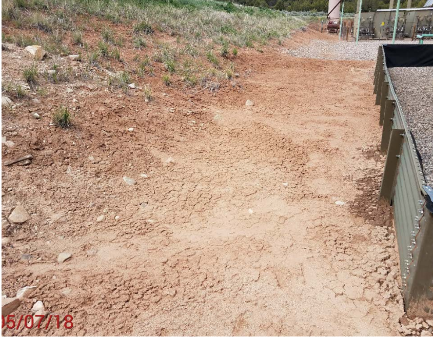
Location photo # 5 storm water erosion on SE corner of Tank Battery
