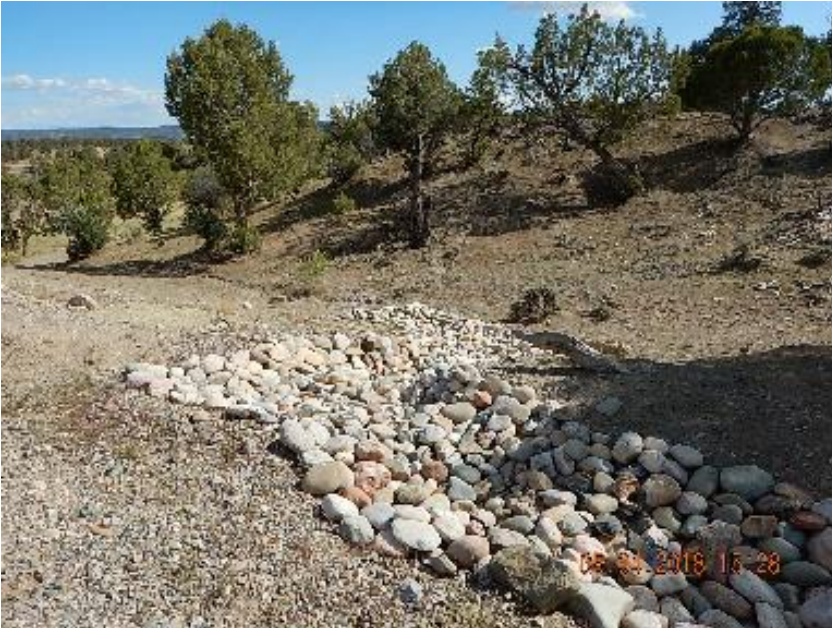
Photo 3: Rock lined drainage heading down slope.
