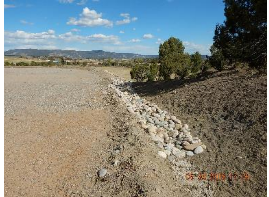
Photo 4: Rock lined ditch on edge of location.
