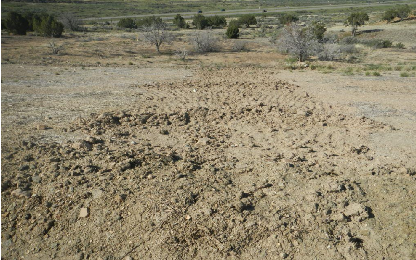
Photo#2: Washed out area in Fill slope has been repaired.
