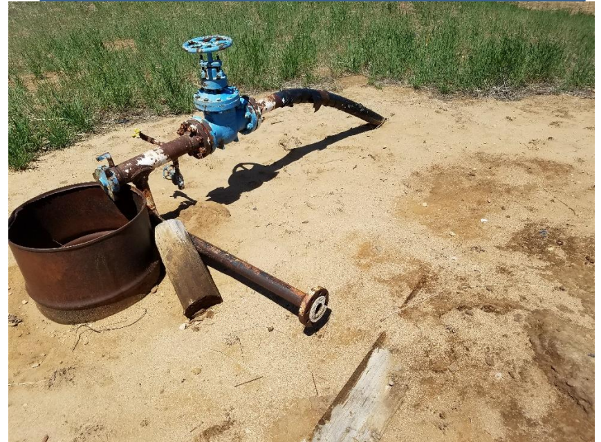
Photo 2. Abandon unmarked riser
