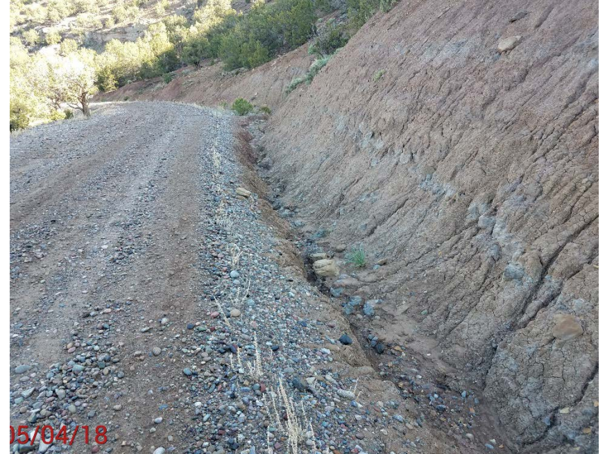
Location photo #2 Ditch erosion along the side of the road
