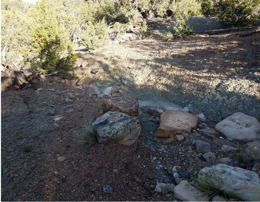
Location photo # 1 Continued Erosion below culvert
