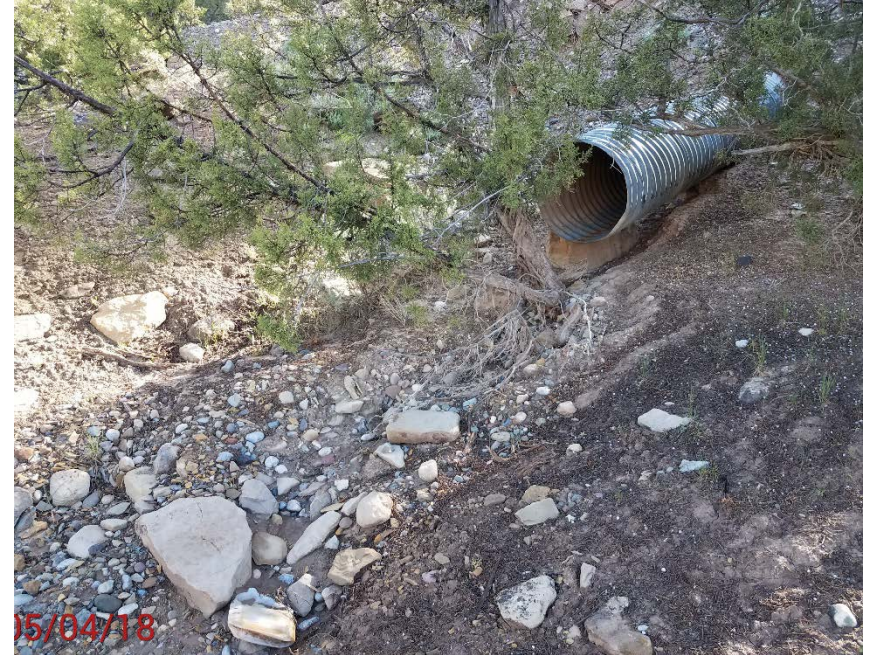
Location photo #2 Erosion at out let of culvert
