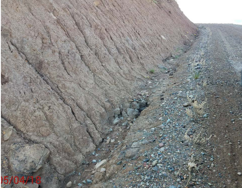
Location photo # 1 Ditch erosion along the side of the road
