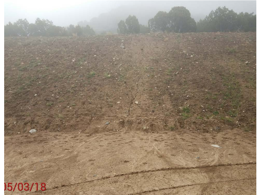
Location photo # 6 slope erosion near separators, looking south
