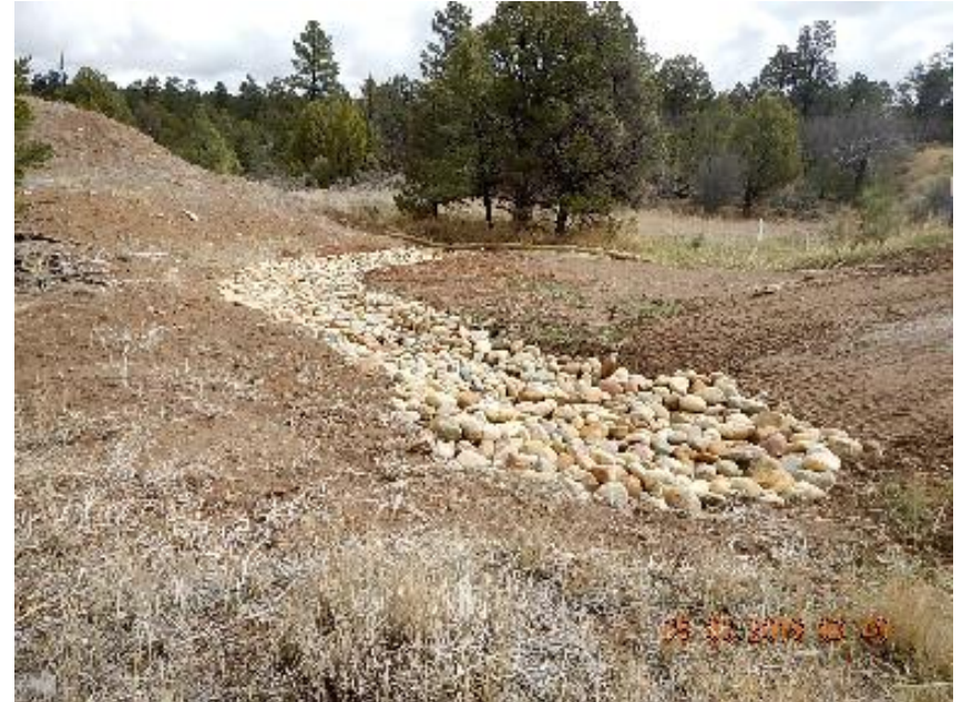
Photo 4: Repaired erosion channel.
