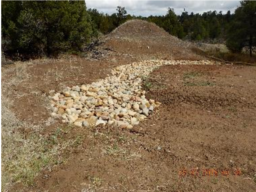
Photo 3: Repaired erosion channel.
