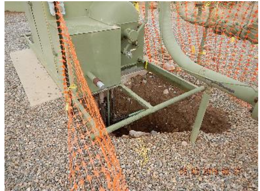
Photo 2: Excavated area at separator to abandon 1" line.
