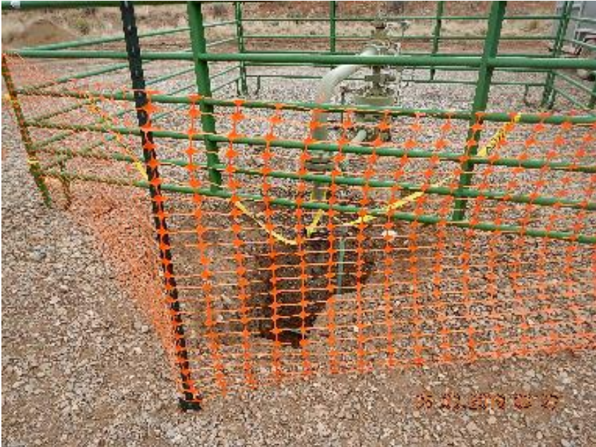
Photo 3: Excavation at wellhead to abandon 1" line.
