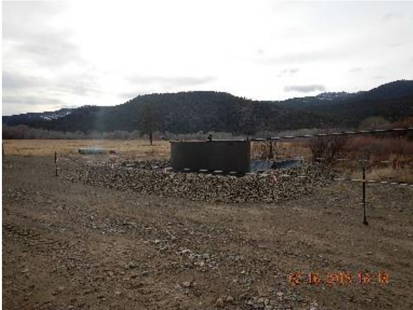
Photo 5: Open top tank with no labels. Previous inspection.
