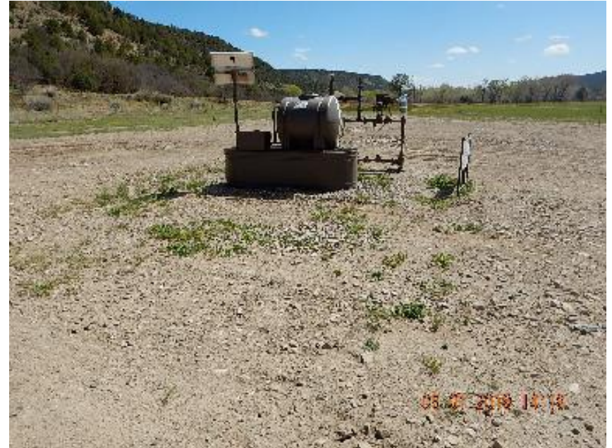
Photo 4: Steel riser removed.
