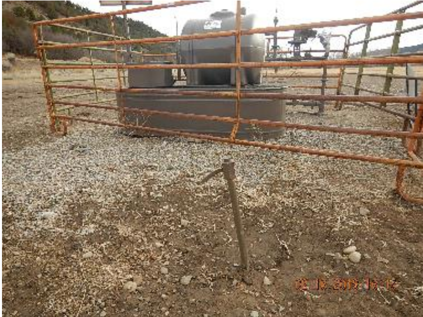
Photo 3: Steel 1" riser outside wellhead fencing. Previous inspection.
