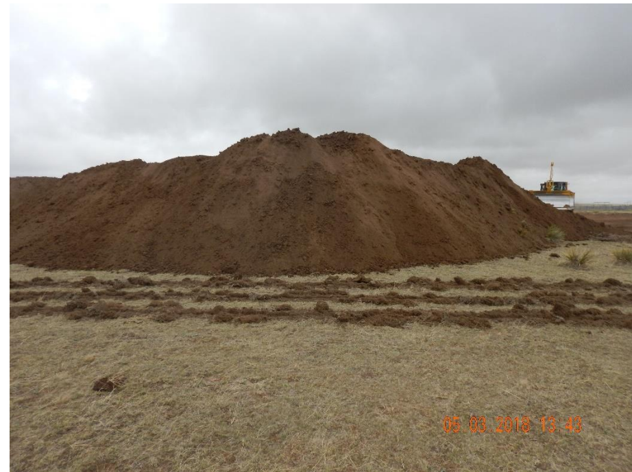
Photo 6: Photo taken from the west end of the construction site. Photo shows topsoil salvage in process. Topsoil will require stabilization.
