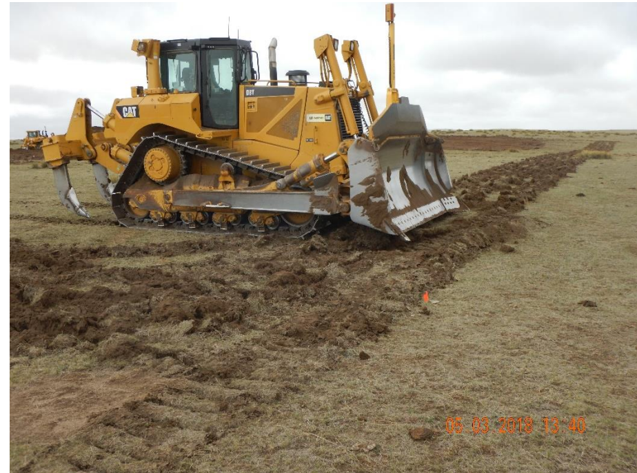
Photo 2: Photo taken from the southeast end of the construction site, facing north. Photo shows operator implemented surface roughening along perimeter of the location. It is noted that surface roughening is a temporary control that should be used in conjunction with other BMPs, and due to ongoing stormwater events, additional BMPs should be considered and implemented. Additional BMPs will need to be installed to replace the surface roughening once the pad has been constructed and stabilized.
