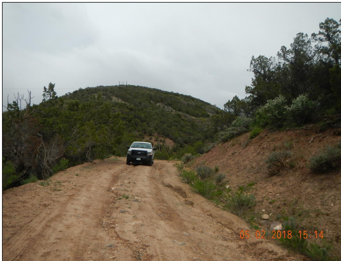
Ruts on access are washing and moving sediment.
