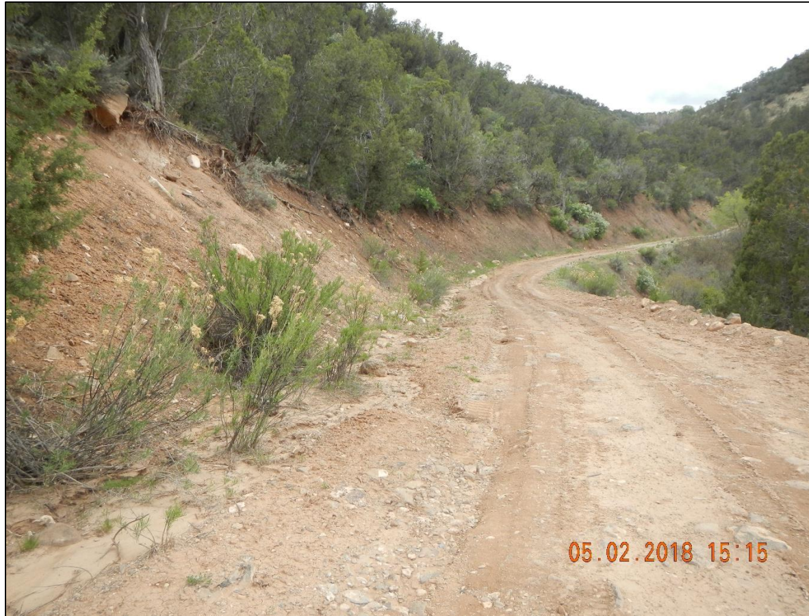
Sediment build up in road ditch.
