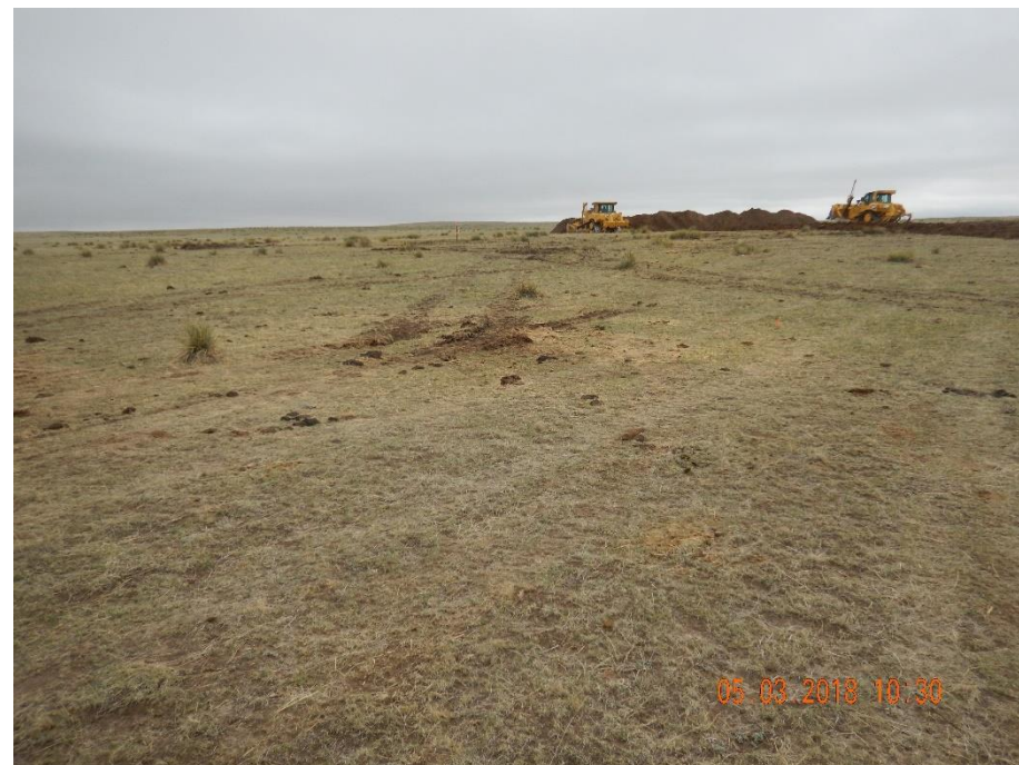
Photo 2: Photo taken from the southeast end of the constructions site, facing west. Photo shows construction activities in process, however, no stormwater and sediment control BMPs have been installed.
