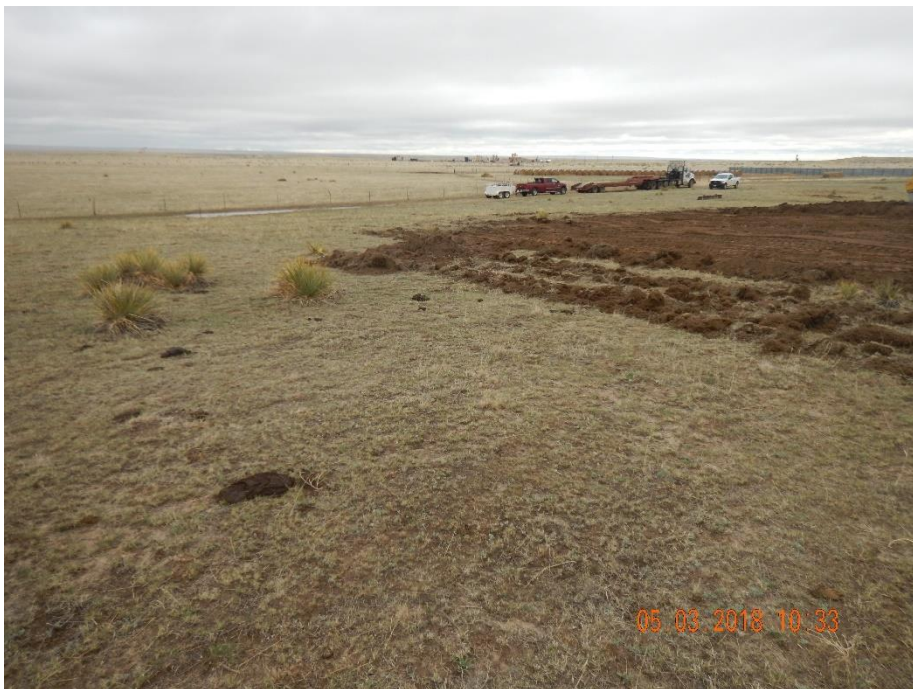
Photo 7: Photo taken from the north end of the construction site, facing southeast. Photo shows construction activities in process, and the topsoil pile however, no stormwater and sediment control BMPs have been installed.
