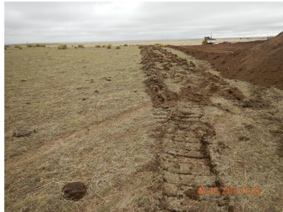
Photo 6: Photo taken from the northwest end of the construction site, facing east. Photo shows surface roughening has been installed on the northern perimeter of the location. Surface roughening alone is insufficient for a control.
