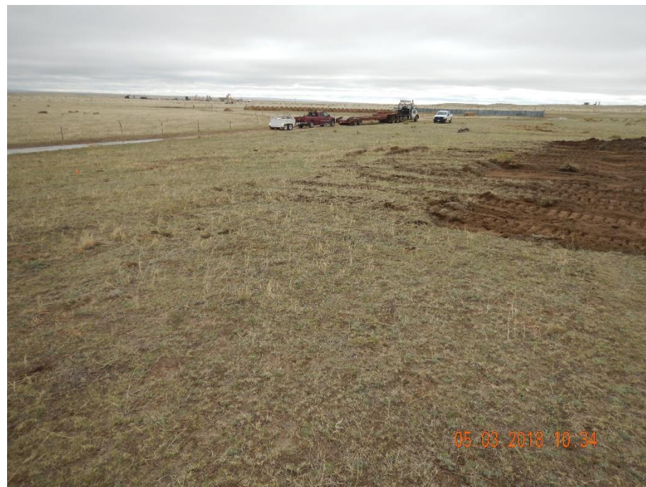
Photo 8: Photo taken from the north end of the construction site, facing southeast. Photo shows construction activities in process, and the topsoil pile however, no stormwater and sediment control BMPs have been installed.
