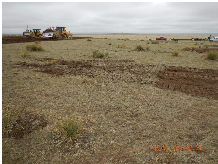
Photo 4: Photo taken from the southwest end of the constructions site, facing east. Photo shows construction activities in process, however, no stormwater and sediment control BMPs have been installed.
