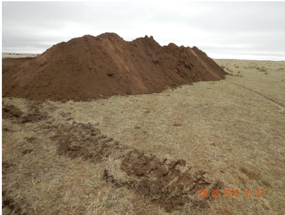
Photo 5: Photo taken from the northwest end of the construction site, facing south. Photo shows construction activities in process, and the topsoil pile however, no stormwater and sediment control BMPs have been installed.
