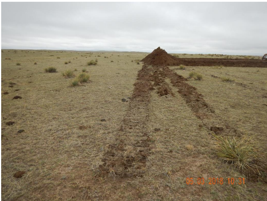
Photo 3: Photo taken from the southwest end of the constructions site, facing north. Photo shows construction activities in process, however, no stormwater and sediment control BMPs have been installed.
