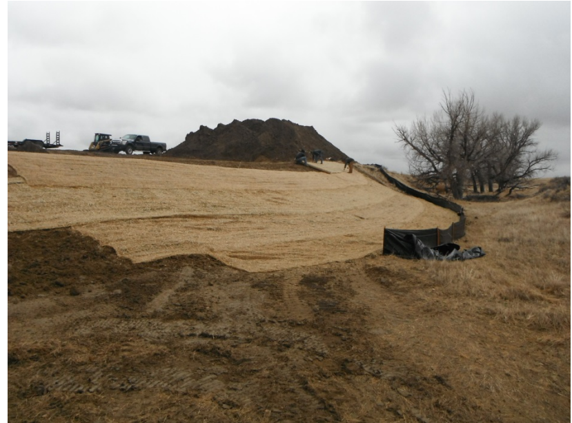
Installation of erosion control blankets
