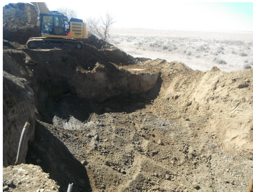
Unimpacted shale in floor of excavation
