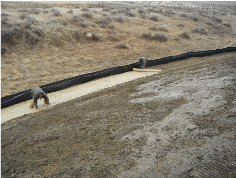
Installation of erosion control blankets
