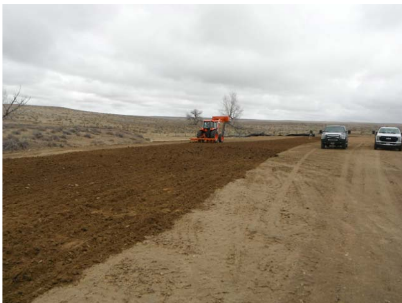
Deep ripping of tank area
