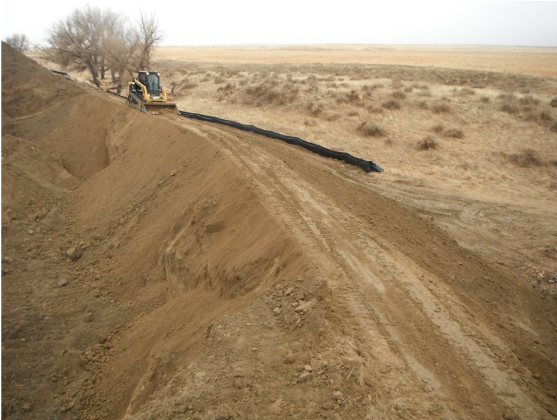
Creating flat surface on top of dike
