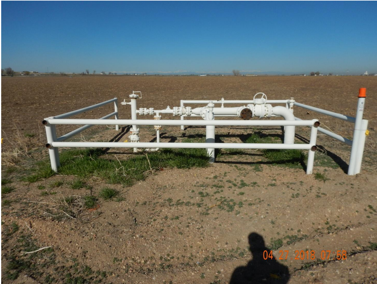
Photo 2. Photo taken of the risers that remain at the location. Operator shall comply with Rule 1004.a.
