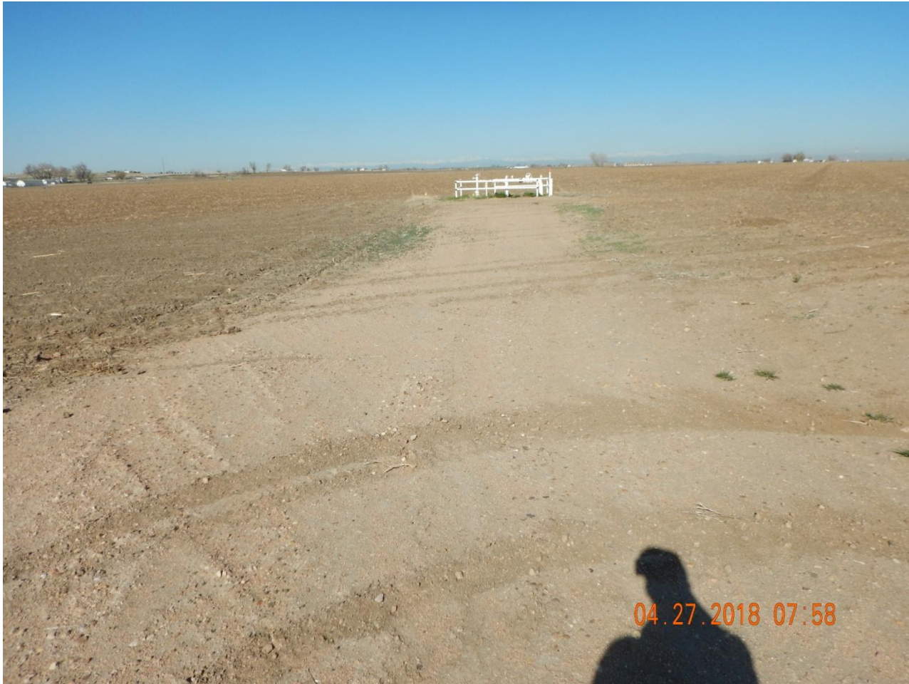
Photo 1. Photo taken from the entrance of the location, facing West. Operator has failed to reclaim a portion of the access road and failed to remove risers from the location per Rule 1004.a.
