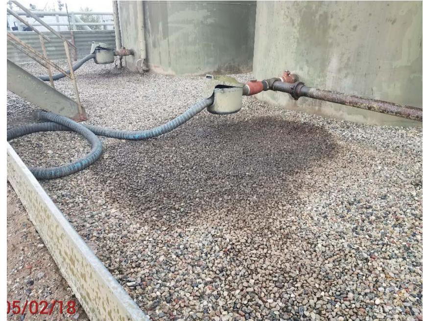
Location photo # 4, Stained material in tank battery containment
