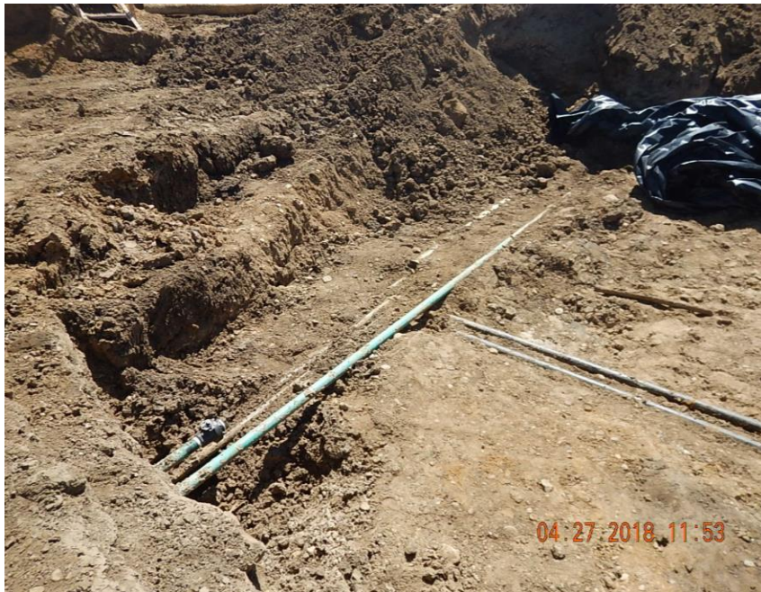
Closer view of flowlines exposed in excavation; The short valved/ plugged line is the active Crude Oil dump flowline (isolated during remediation); and (4) historically abandoned flowlines. Note: Photo taken 4/27/18
