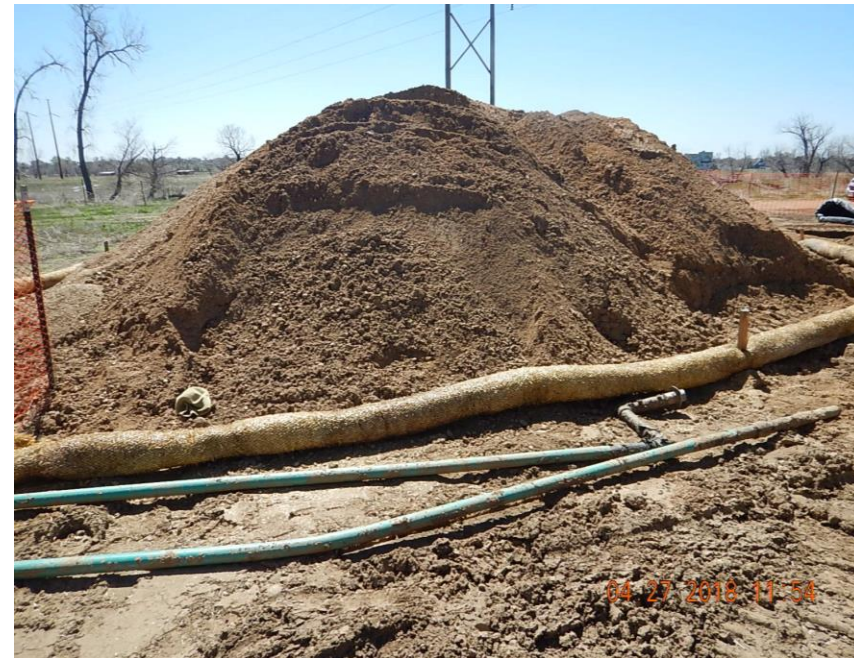
Waddles surrounding soils stockpile and flowline pipe materials removed from excavated area.
