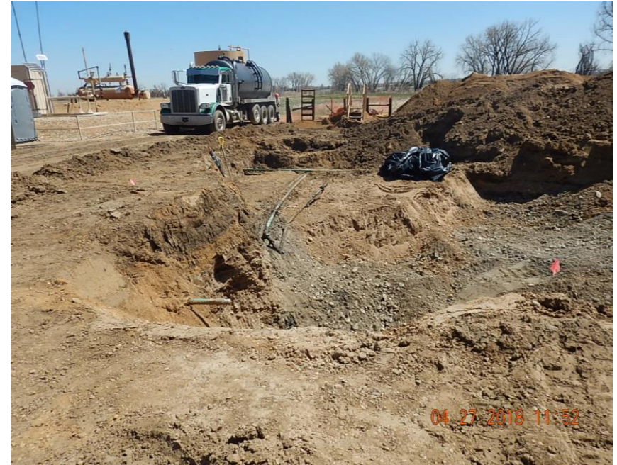
Closer view of excavated area exposing both active dump lines and (previously unknown) historically abandoned flowlines (view to East) Note: Photo taken 4/27/18
