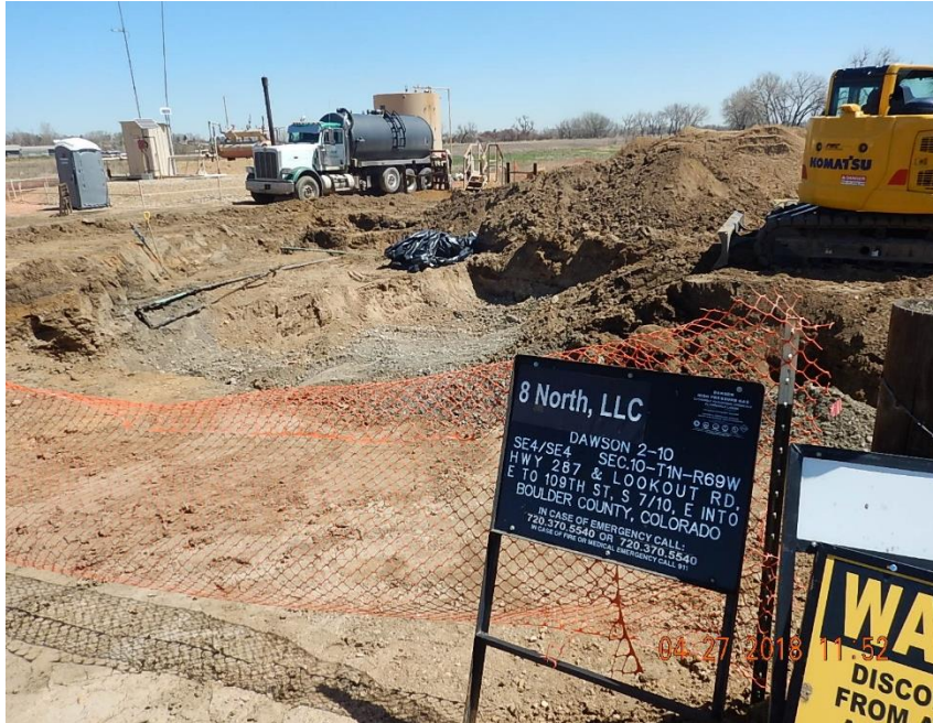
Location signage and view of phase 1 remediation area on location. Flowlines are exposed in the excavation (view East) Note: Photo taken 4/27/18
