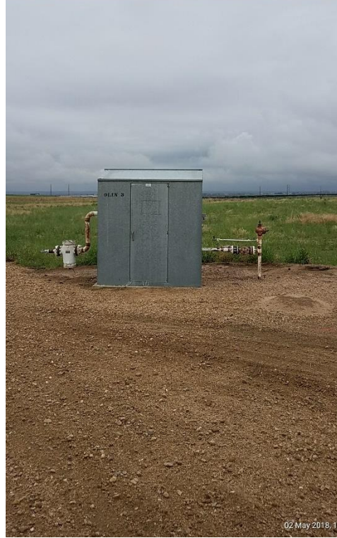
Photo 5 Disconnected GMR
