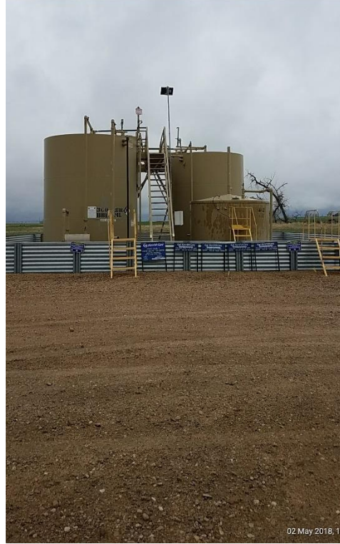
Photo 2 Tank Battery
